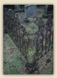
The iron is extremely corroded and rusted.
