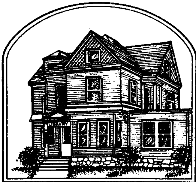
Brigham House in Newton Highlands
