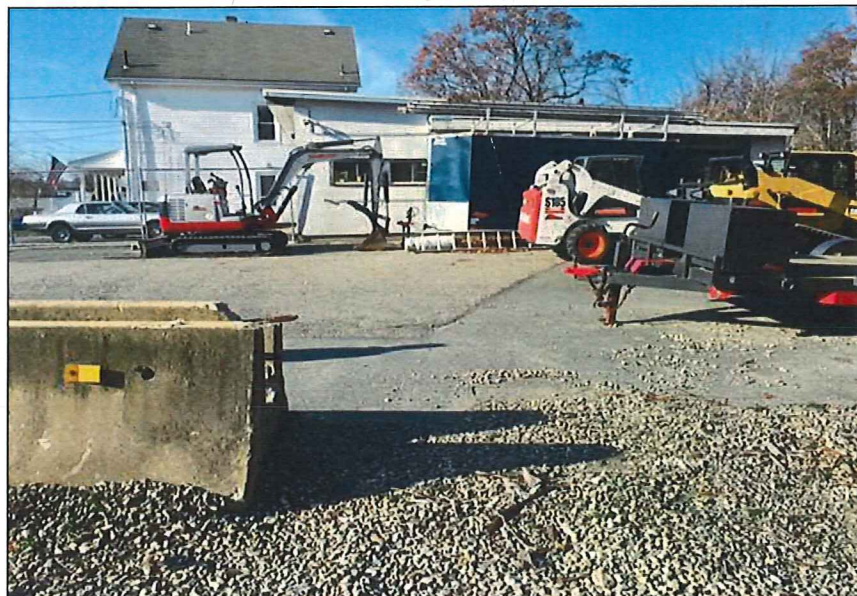
Figure 5. Note areas of pavement in vicinity of garage.
