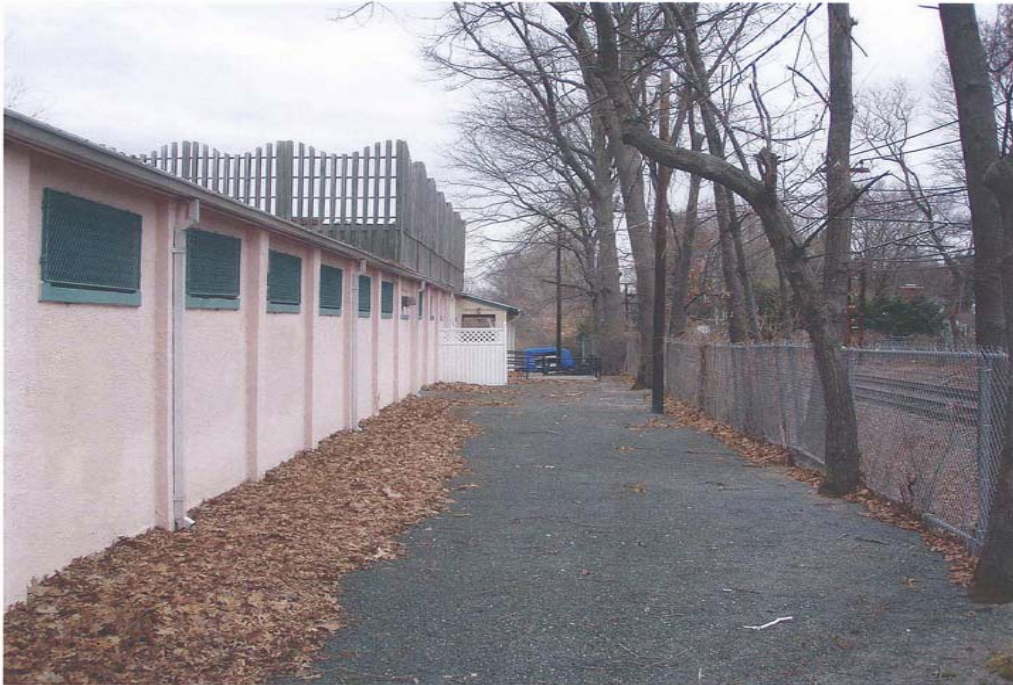
Figure 10: Rogers St. View of MBTA Side of Bathhouse
