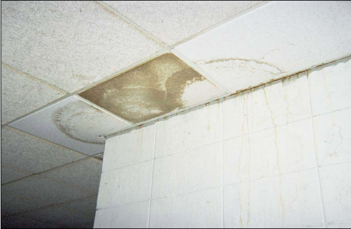
Figure 18: Interior Bathhouse - Ceiling Tiles
