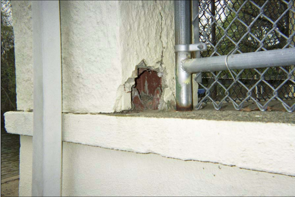
Figure 12: Original Building- Stucco Over Clay Tile Block
