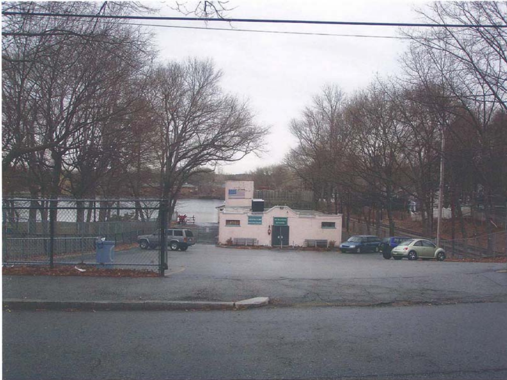
Figure 6: View of Bathhouse and Parking Lot from Rogers Street
