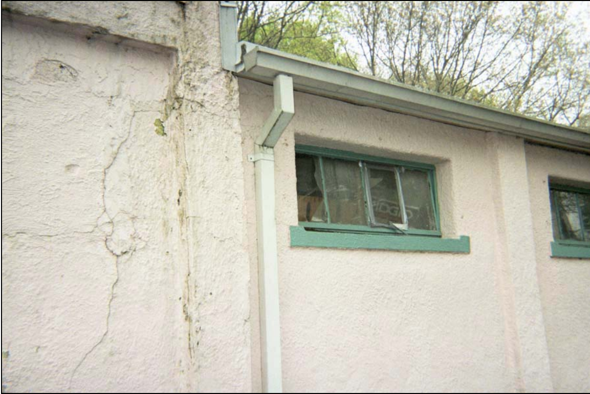
Figure 16: Exterior Bathhouse - Windows, Stucco and Roof Drainage
