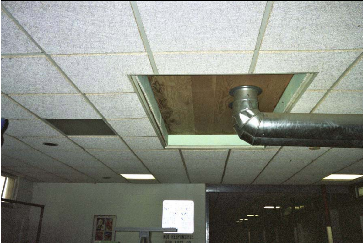
Figure 26: Interior Bathhouse - Ceiling
