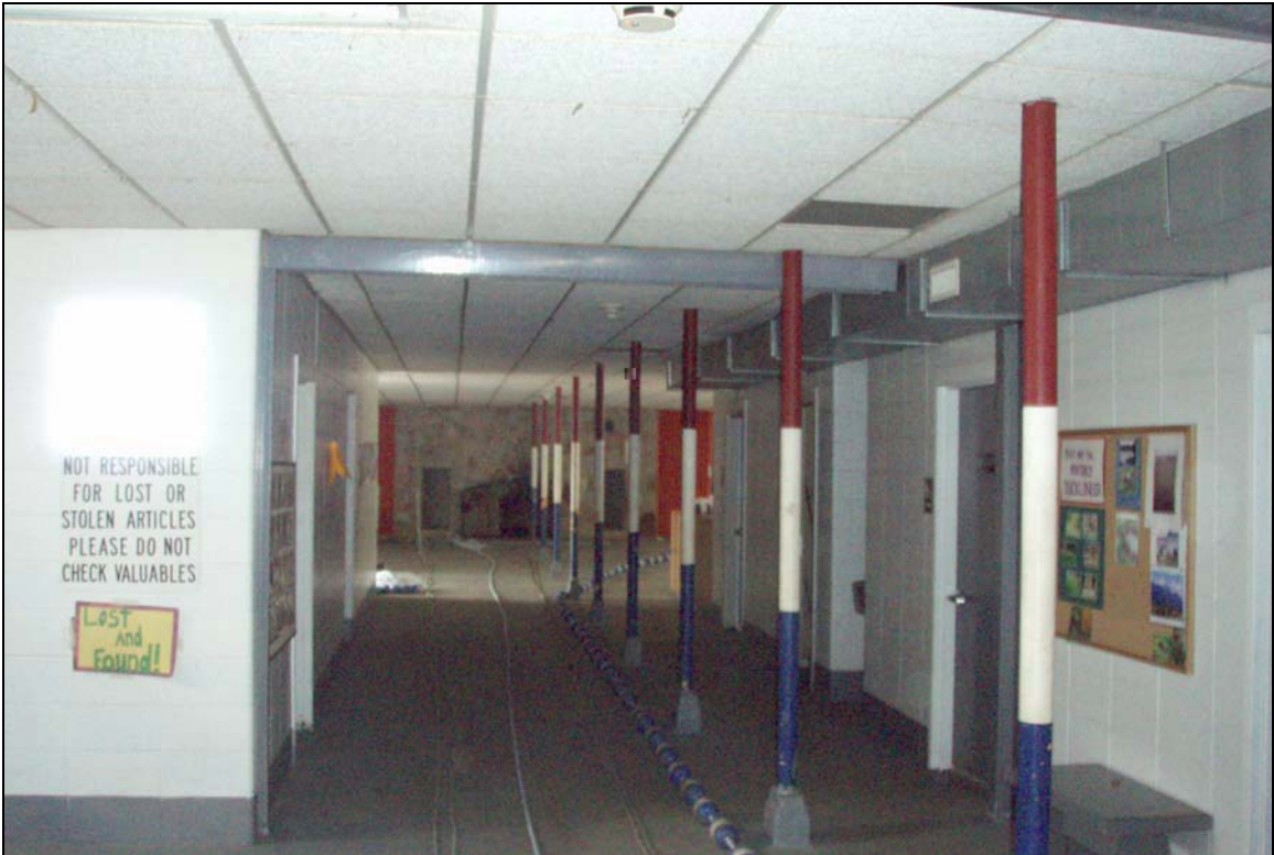
Figure 27: Interior Bathroom - Corridor Leading from Front Desk to Fireplace
