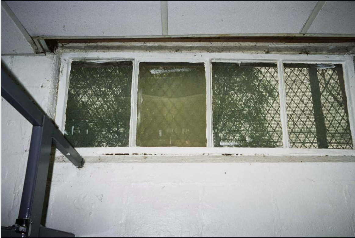
Figure 24: Interior Bathhouse - Windows
