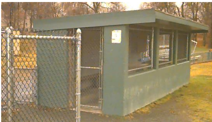
Dugout on ball field in Lyons Park, Auburndale
