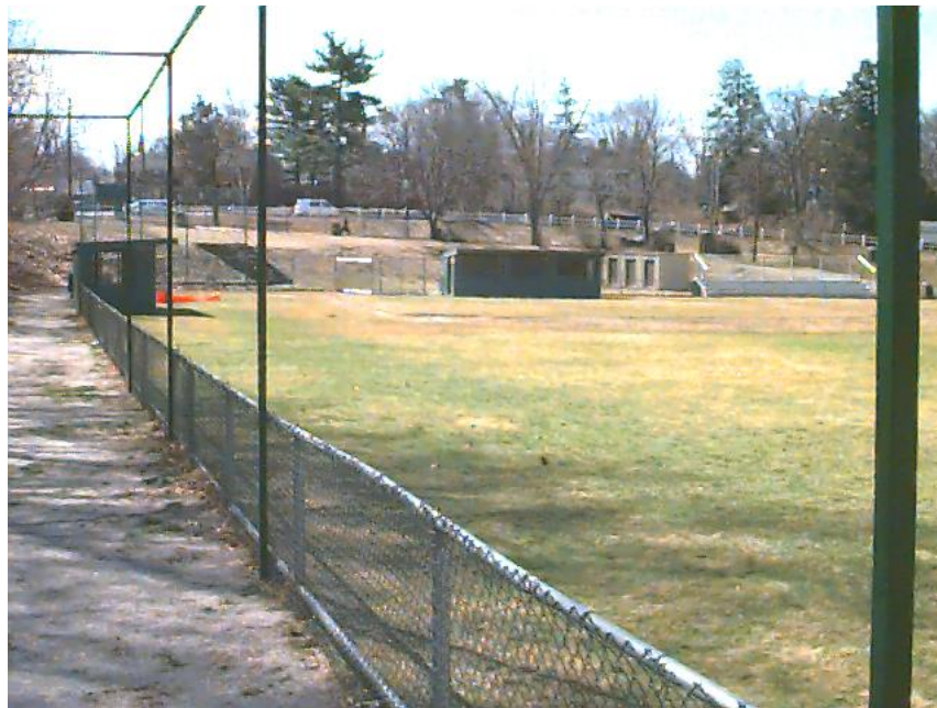
Fences, Batting Cage, Dugouts and Grandstand, Lyons Park
