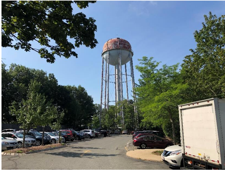
View of subject from parking lot adjacent to Stanton Avenue
