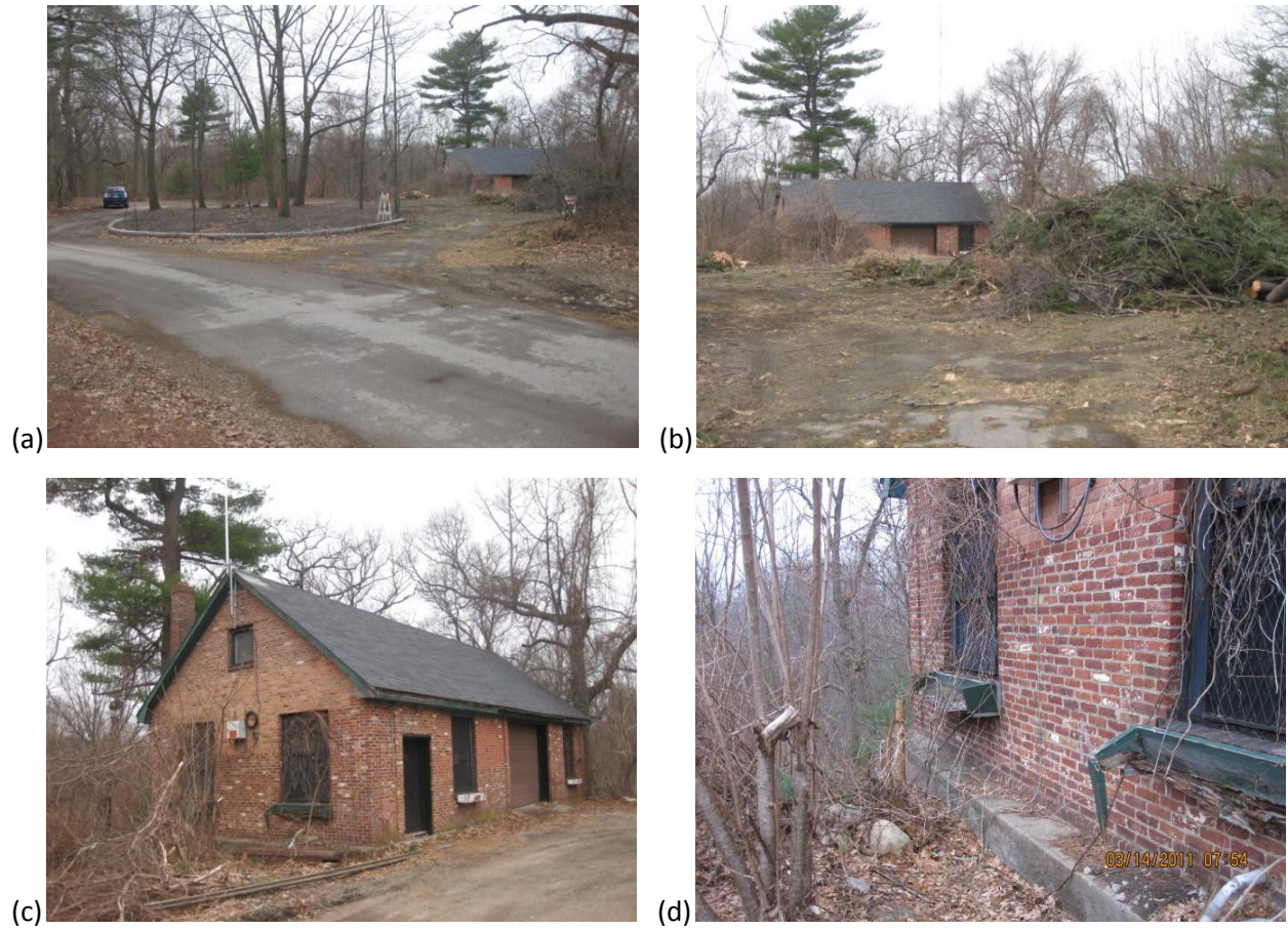
Figure 12. Utility lot (a) viewed from Winchester Street entrance, (b) with brush pile on 4/11/11. A view (c) of the brick building and (d) unkempt exterior.
