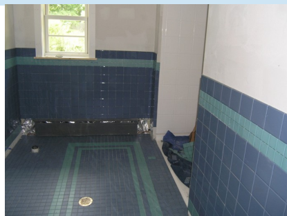
After ADA-complaint bathroom
