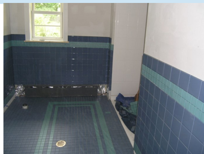
After ADA-complaint bathroom
