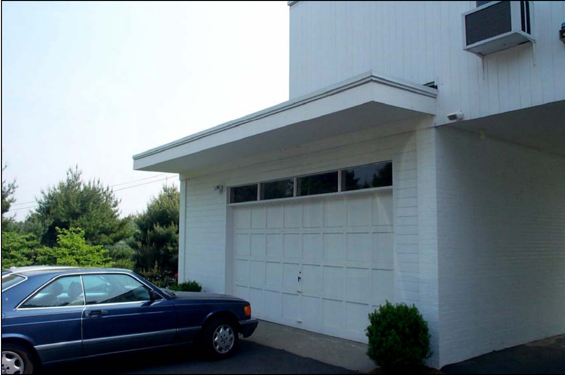
View of Garage from Driveway
