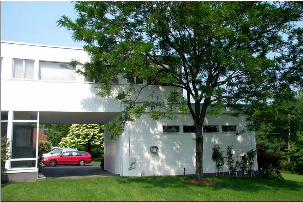
View of Garage Facing Dudley Road
