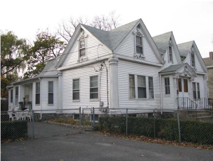
Front / South facade
