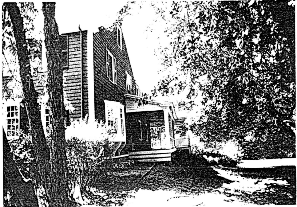
North side looking west
