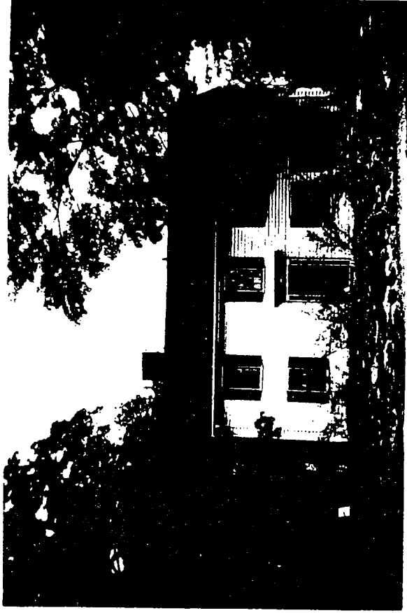
7. SOUTH FACADE WITH SHUTTERS (1962)
