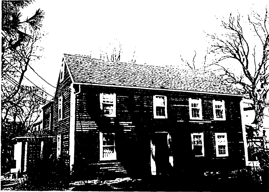
1. SOUTH FRONT FACADE
