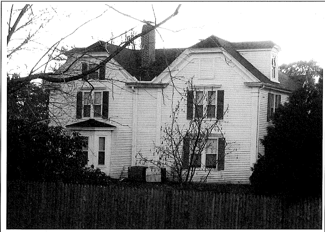
1615 Beacon Street, front façade, view from east looking west
