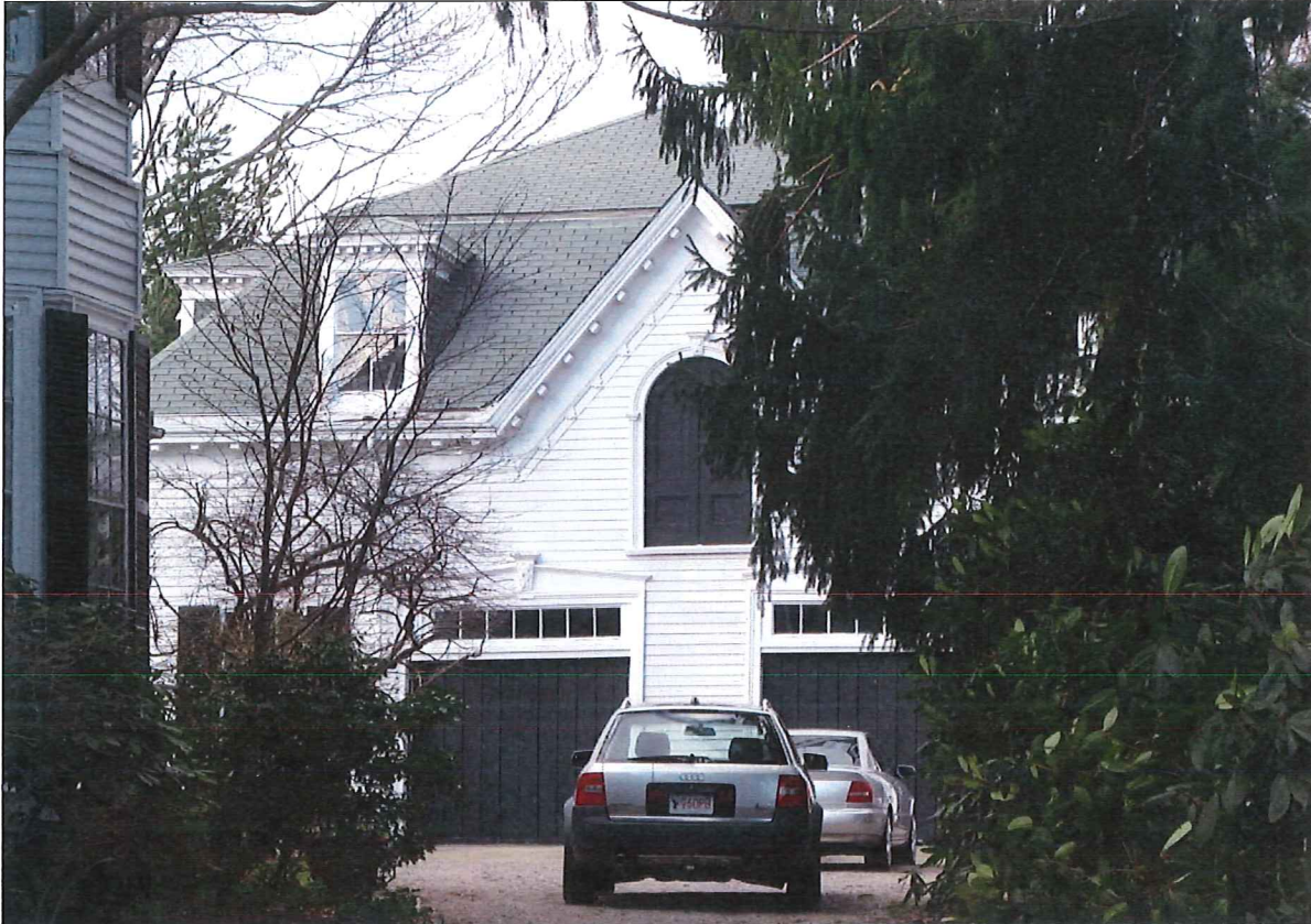
View of barn from south
