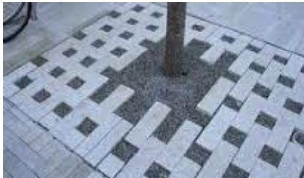
CONCRETE PAVERS ON STRUCTURE AT TREE WELLS
