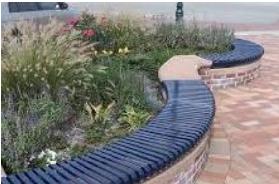
PRECAST CONCRETE SEATWALL
