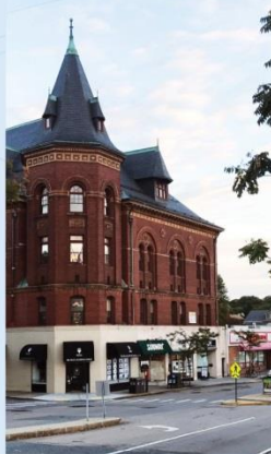
Masonic Building in Newtonville
