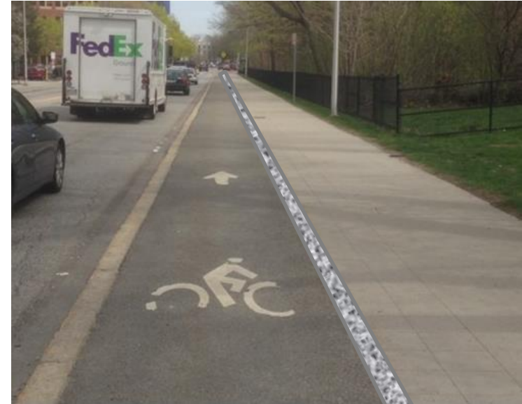
EXAMPLE of raised bike lane
