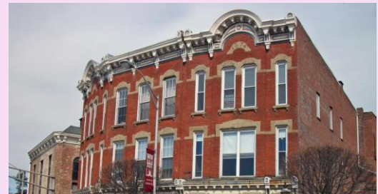
Shape the roofs of buildings
