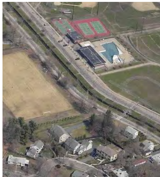
Aerial image showing the angled parking along the east side of the corridor at Albemarle Park and Gath Pool. Cheesecake Brook forms the dark linear form near the center of the photo. To the west of the Brook the roadway width is limited with restricted parking and no sidewalk.
