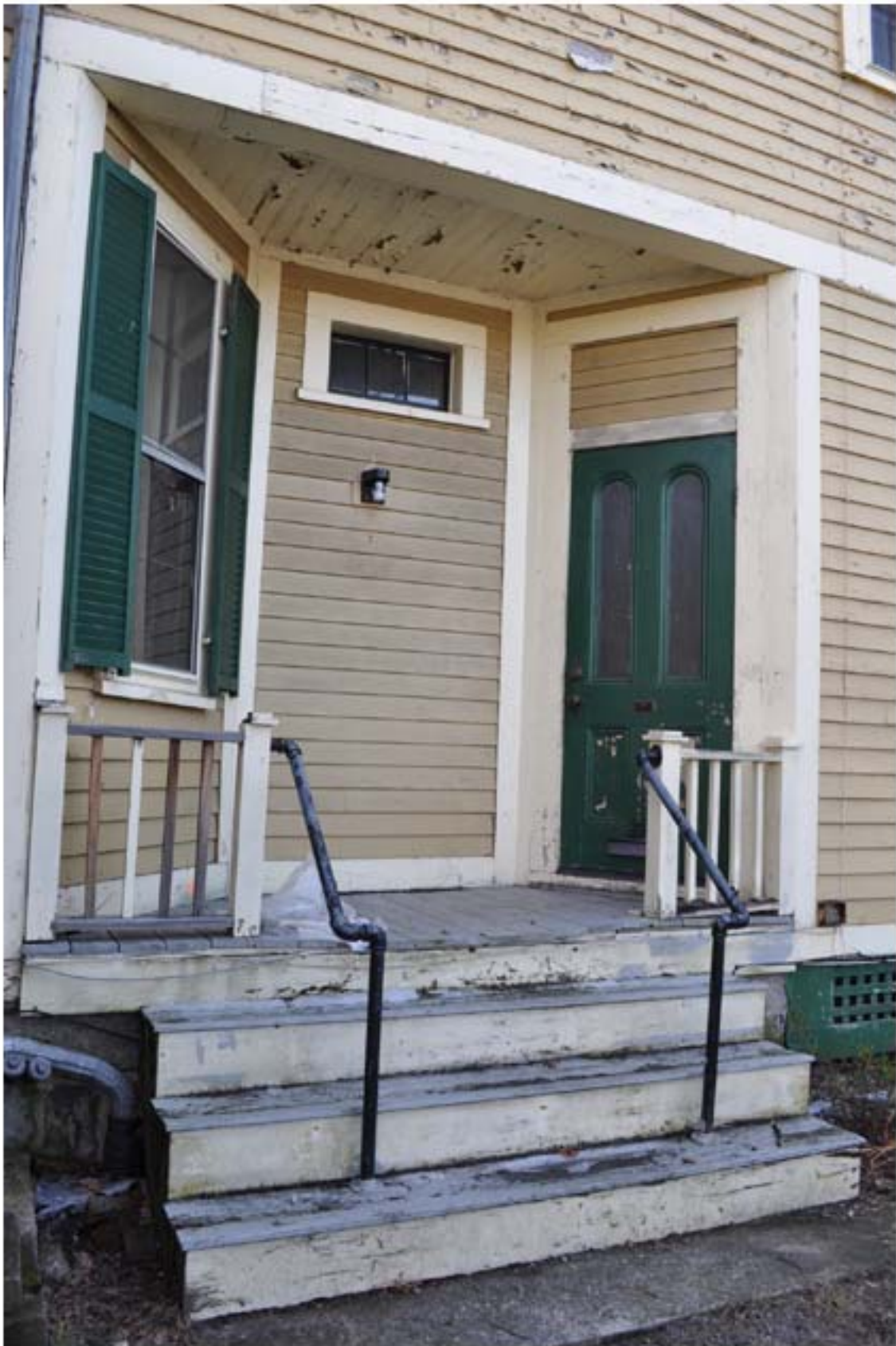
16B- Existing wood porch and steps on west side of house
