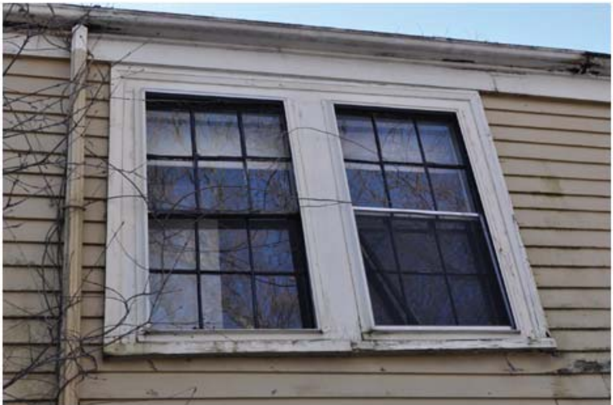
12D- Existing window trim
