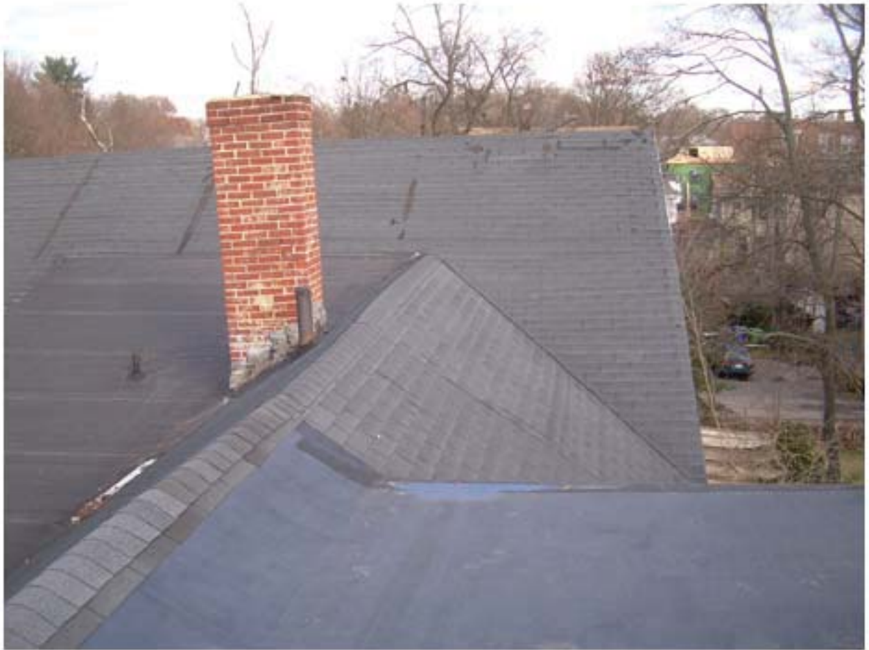
6A- Existing barn chimney
