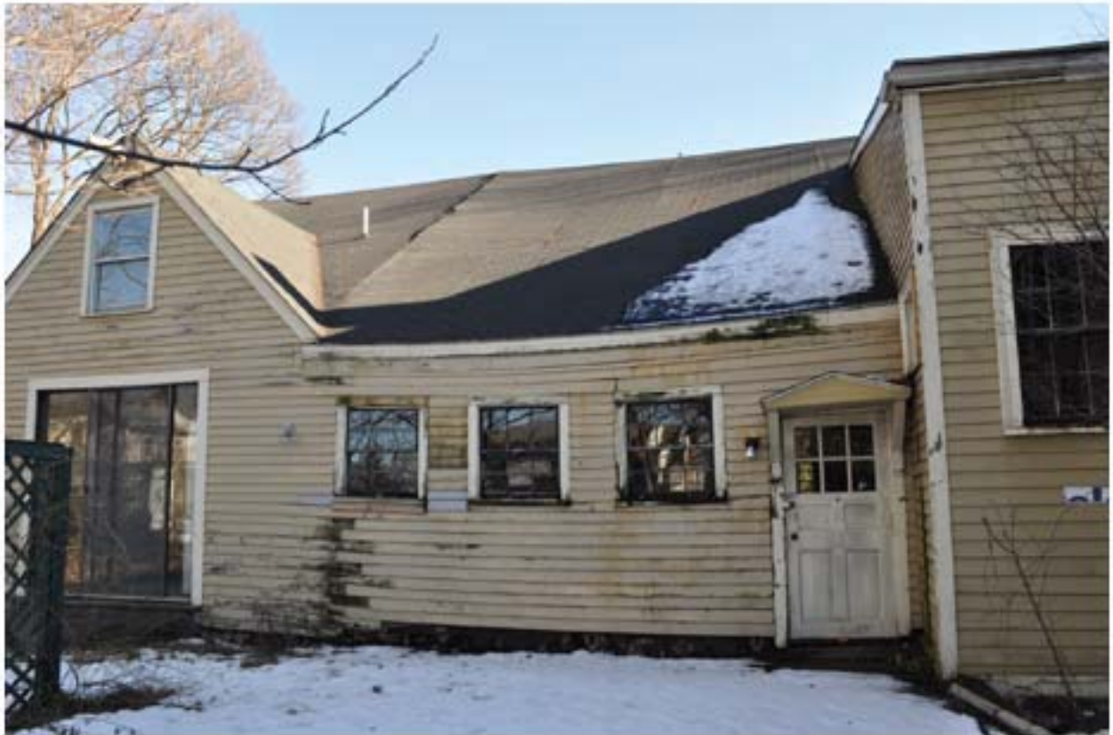
21A- Existing west side of barn
