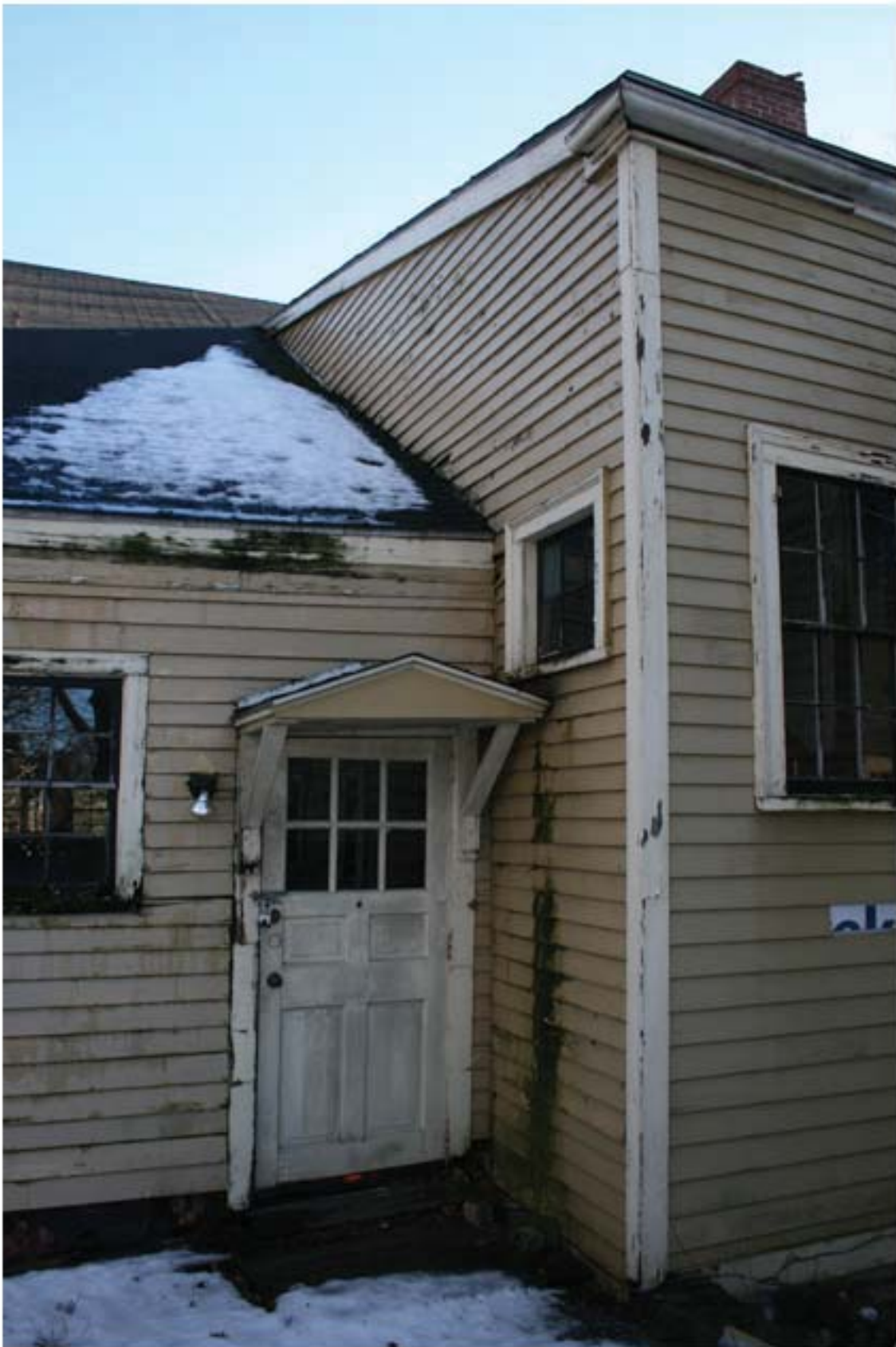
15E- Existing west barn entrance door
