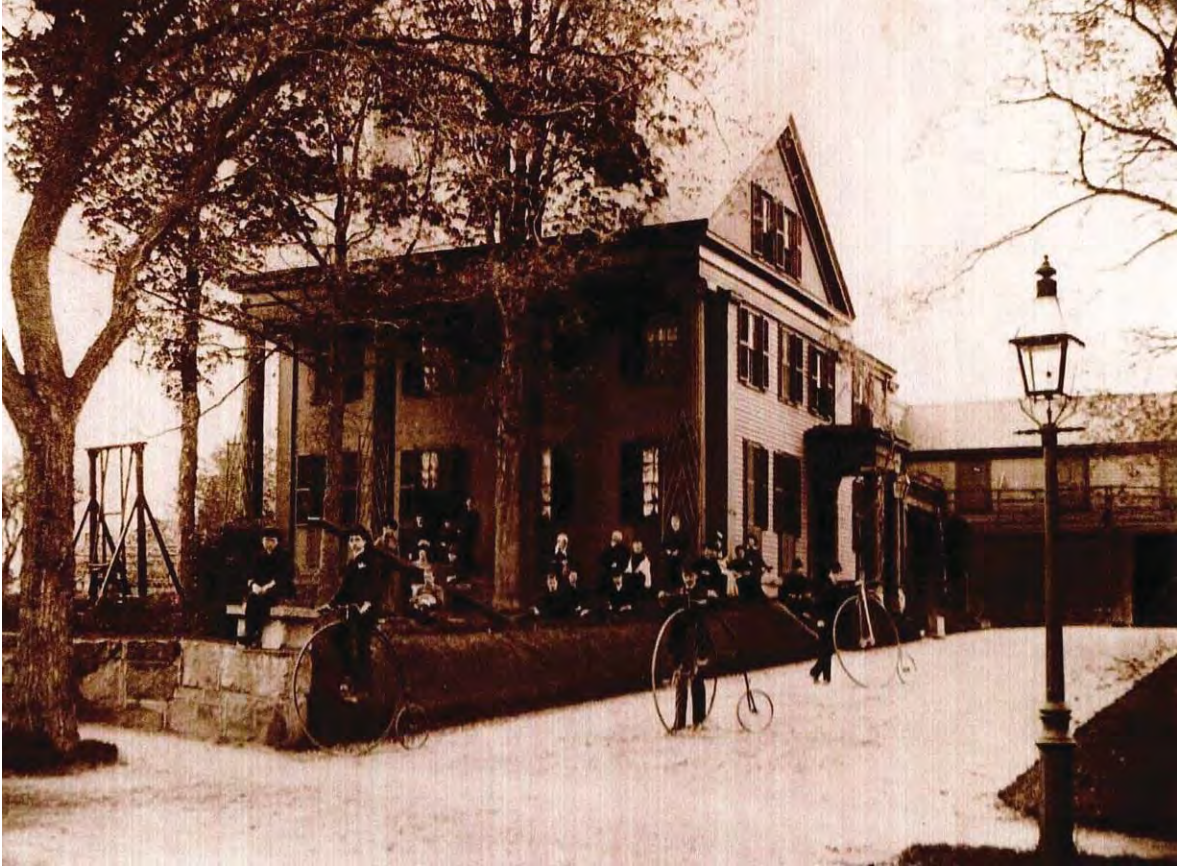
Nathaniel Allen House, Description of Rehabilitation
