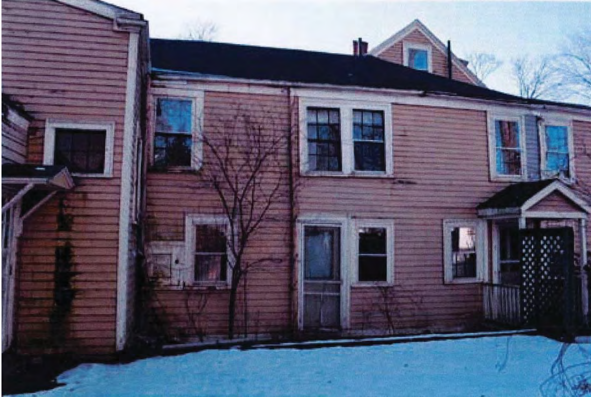
Nathaniel Allen House, Description of Rehabilitation
