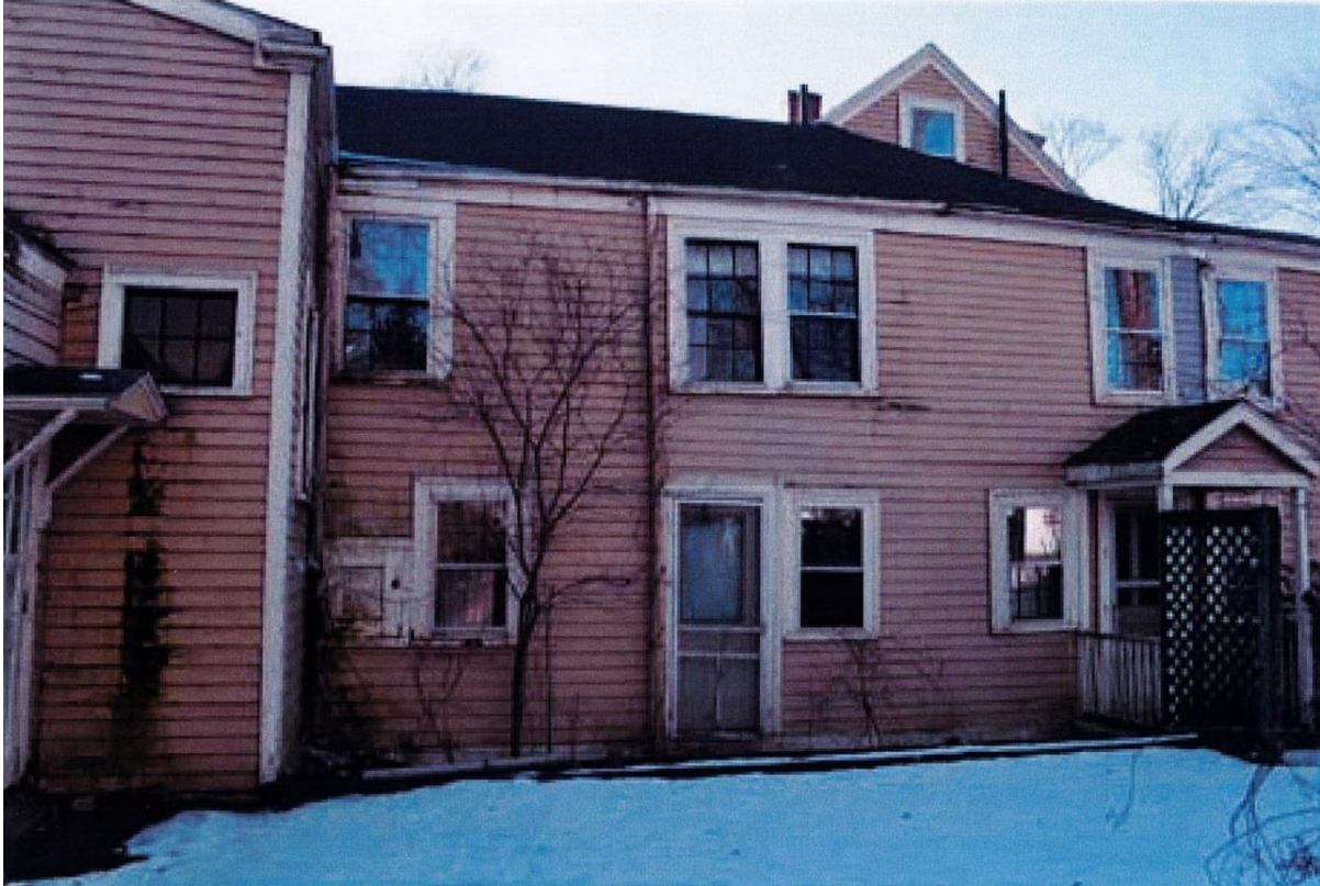
Nathaniel Allen House, Description of Rehabilitation
