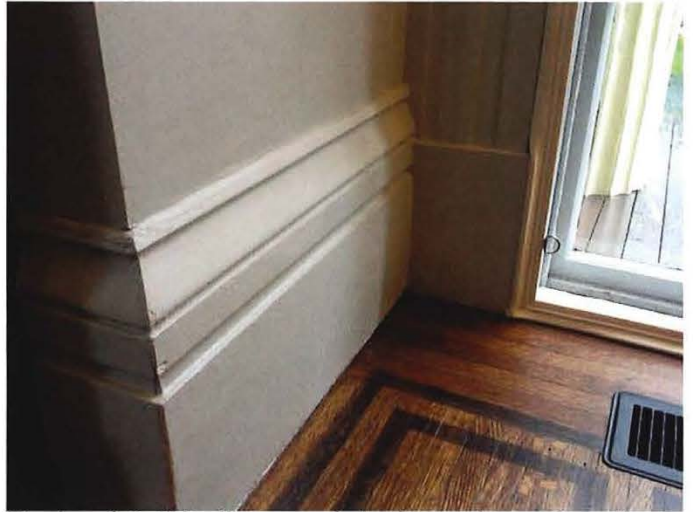
Parlor 1 tall built up painted mopboard and window trim
