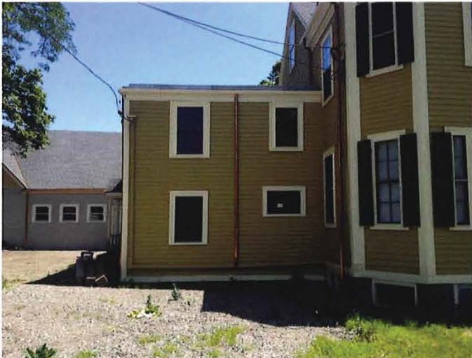
Two Story North Side Ell (West)
