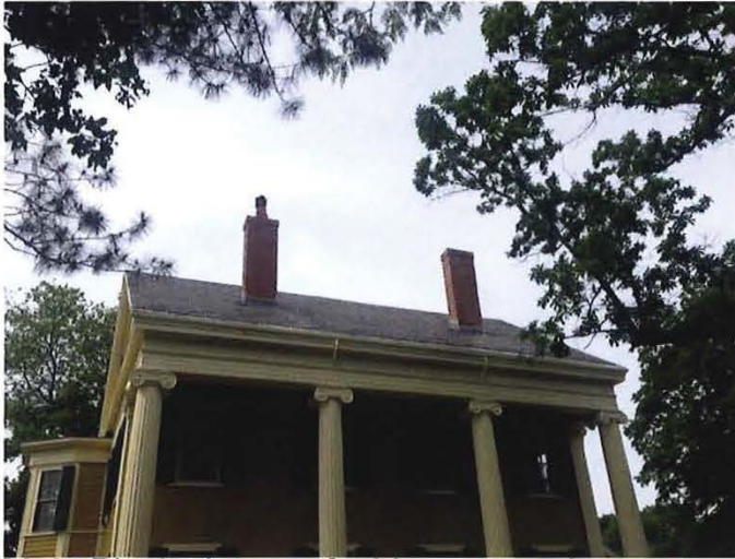
Main Block slate roof, chimneys and chimney pot facing South
