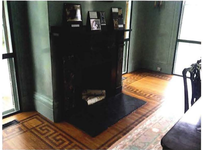
Parlor 2 fireplace surround and mantle
