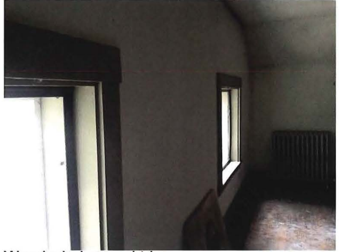
Wood window and trim
