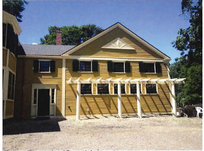
Barn Facade (South)
