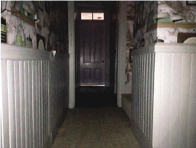
Service Stair Hall base boards and wainscot trim
