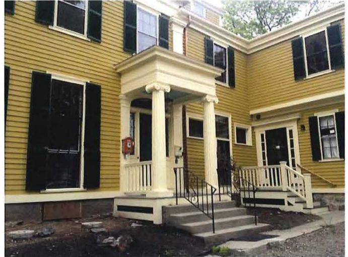
East side Main Entrance Porch w/ roof, cornice, columns, doors and leaded glass sidelights
