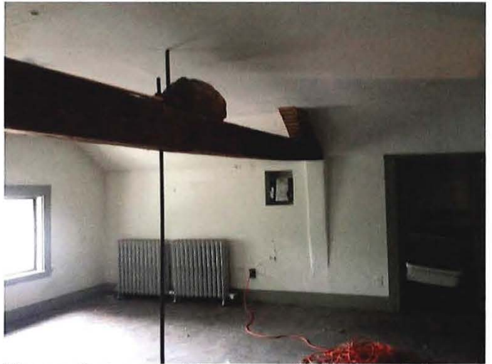
Heavy timber roof trusses with iron rods in Science Classroom
