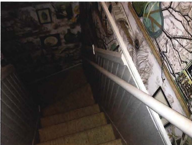
Service Stairway handrail, stair board and wainscot trim
