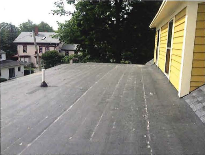
West Side Ell flat roof and dormer
