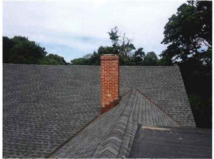
Asphalt roof and chimney facing Northwest
