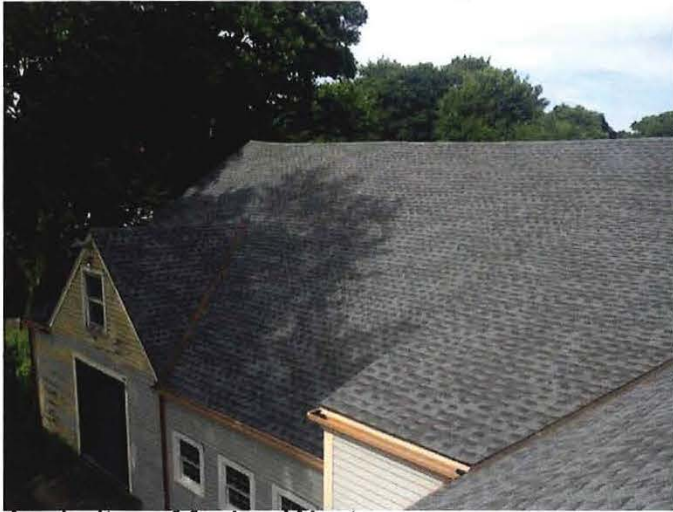
Asphalt roof facing West
