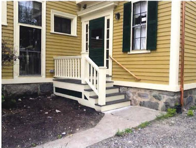
Side Open Porch on the East side
