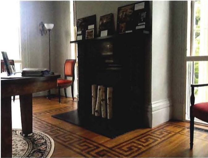
Parlor 1 fireplace surround and mantle
