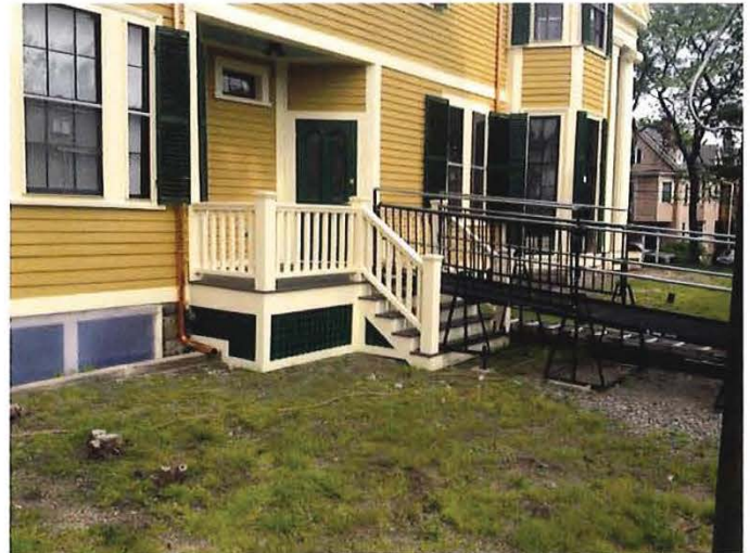
West side Recessed Entrance Side Porch (Temporary HC ramp until main accessible entrance is added in future phase)
