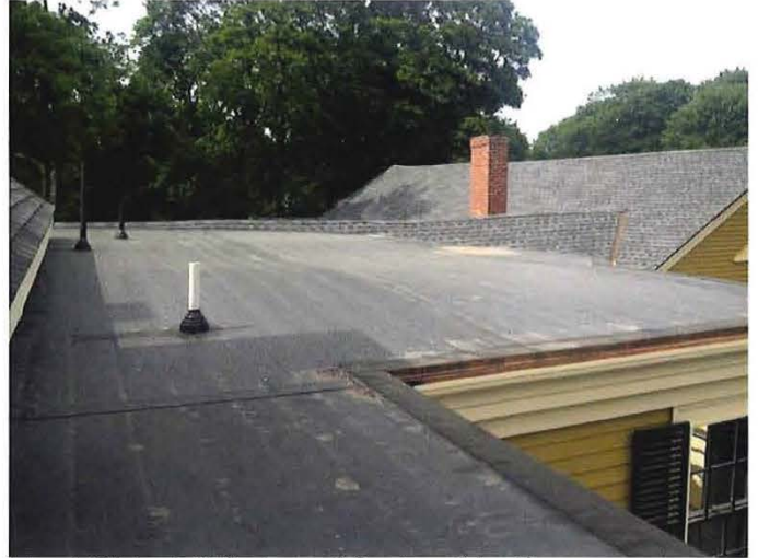
East Side Ell flat roof facing North
