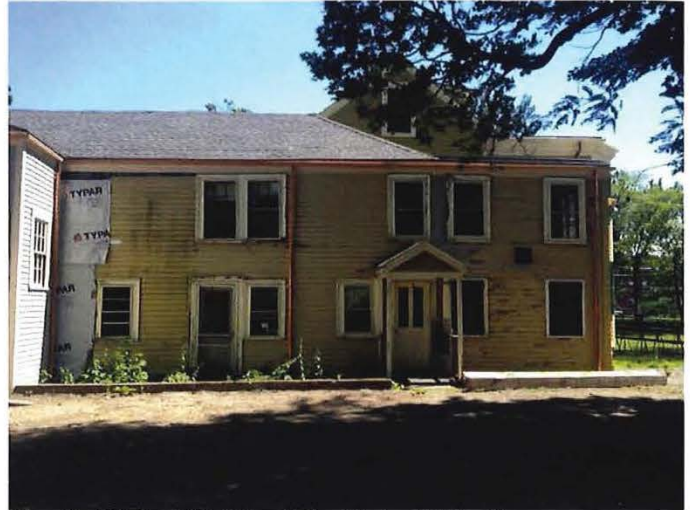
North Side Ell (North)- Rehabilitation scheduled for future phase
