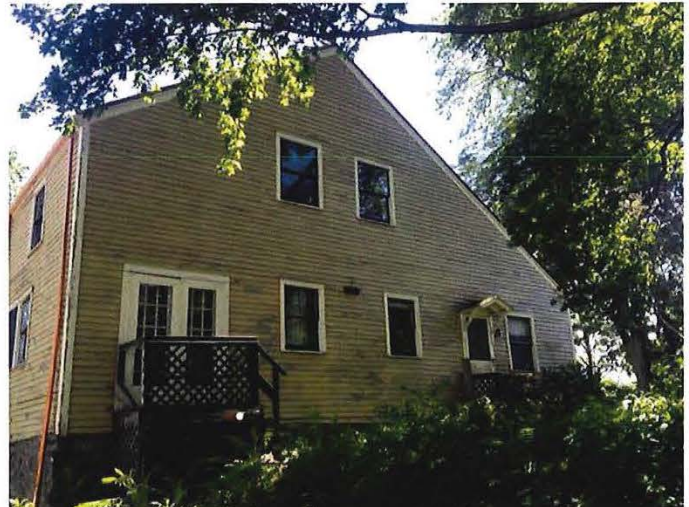
Barn (North)- Rehabilitation scheduled for 49 future phase
