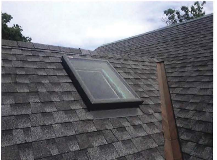
Rear Ell historic skylight facing West
