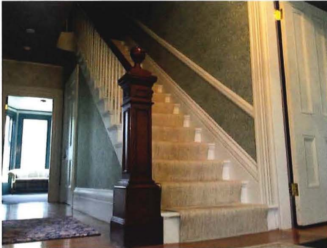
Main Entrance Stairway, newell post, handrail, balusters, stair board and trim
