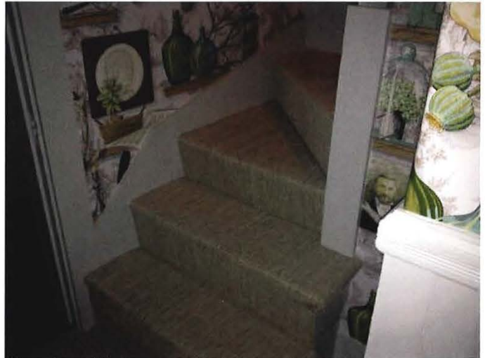
Service Stairway stair board
