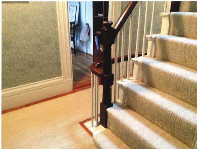
Second floor Main Entrance Stairway newell post, handrail and balusters
