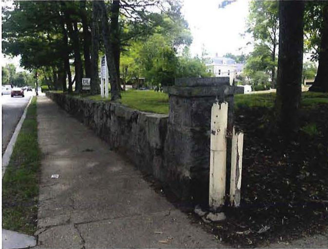
Large square granite post at driveway connecting to low dry laid stone retaining wall along Webster Street public sidewalk
