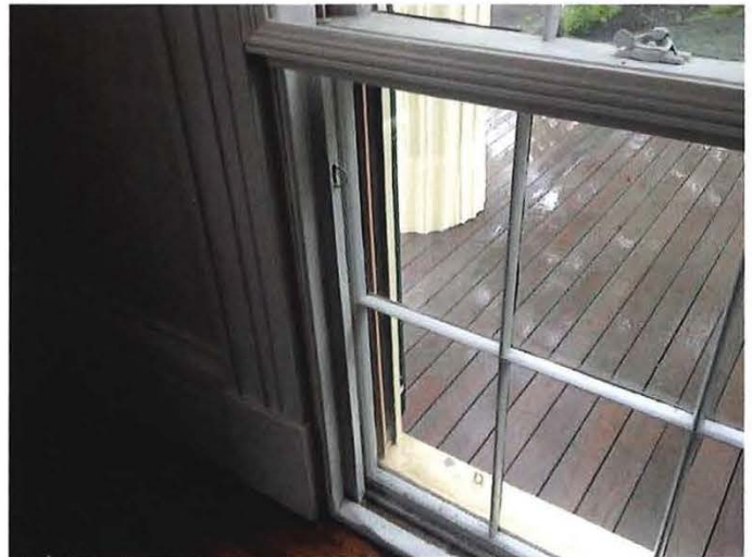
Parlor 1 recessed window shutters
