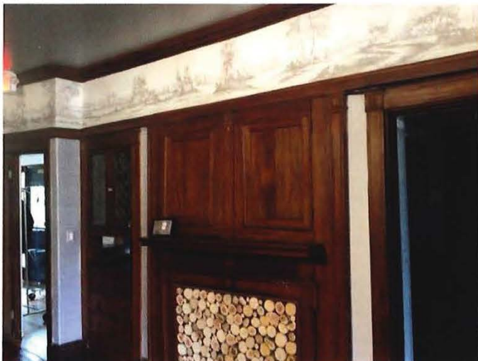
Plate rail and fire place trim
