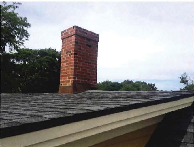
Rear Ell asphalt dormer roof and chimney facing West
