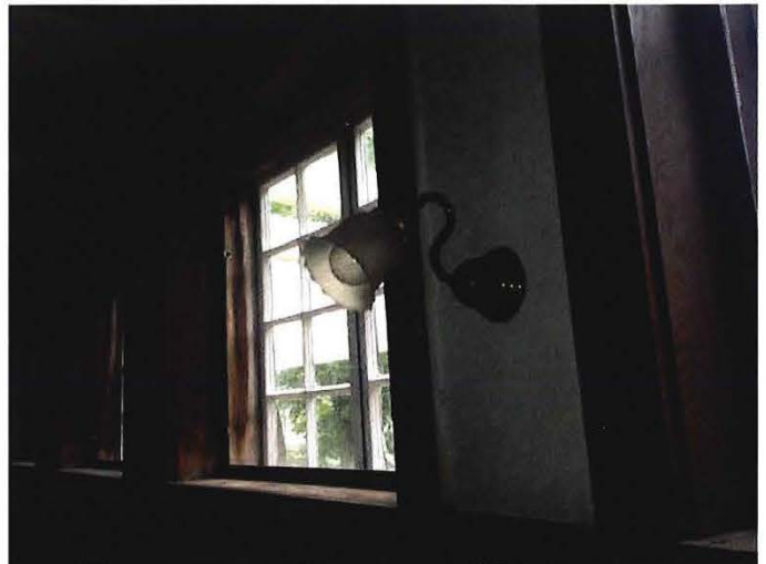
Electrified gas wall sconce light fixture
