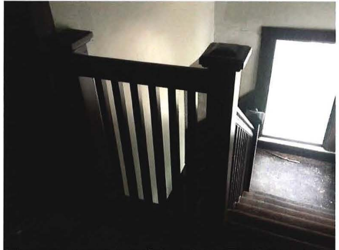
Stairway newell post, handrails and balusters
