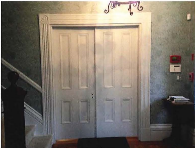
Main Entrance Hallway four panel door, plinth block, fluted door casings and corner block trim
