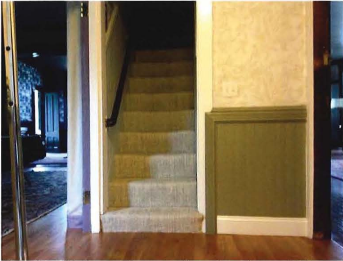
Service Stairway handrail and wainscot trim
