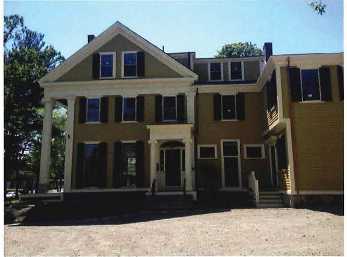
Main House (East)
