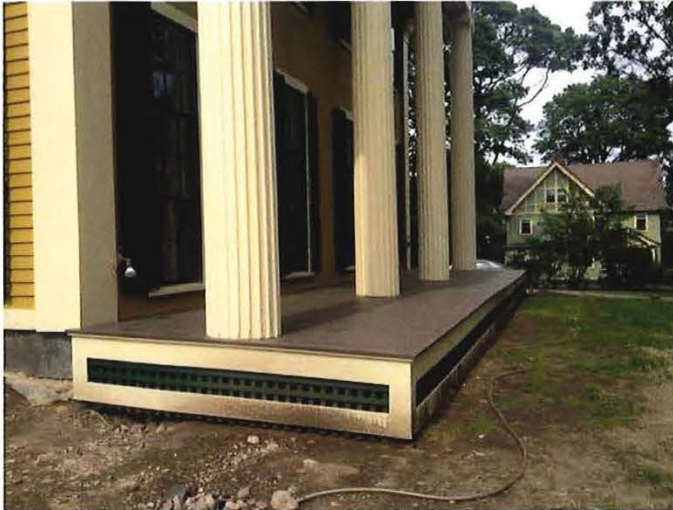
South side Porch including four monumental ionic columns facing Webster Street
