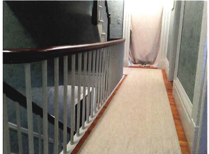
Second floor Main Entrance Stair Hall hand rail and balusters
