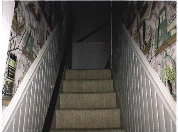
Service Stairway handrails, stair boards and wainscot trim
