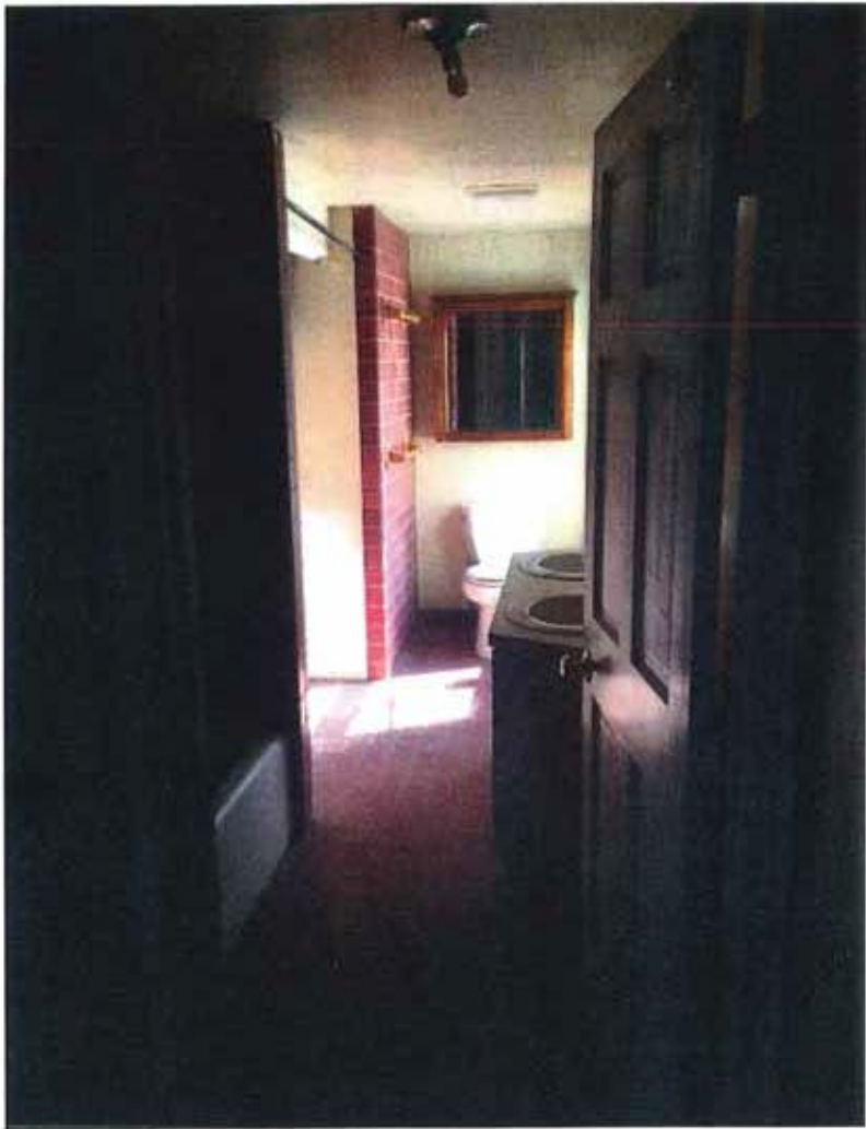
VIEW OF EXISTING BATHROOM
