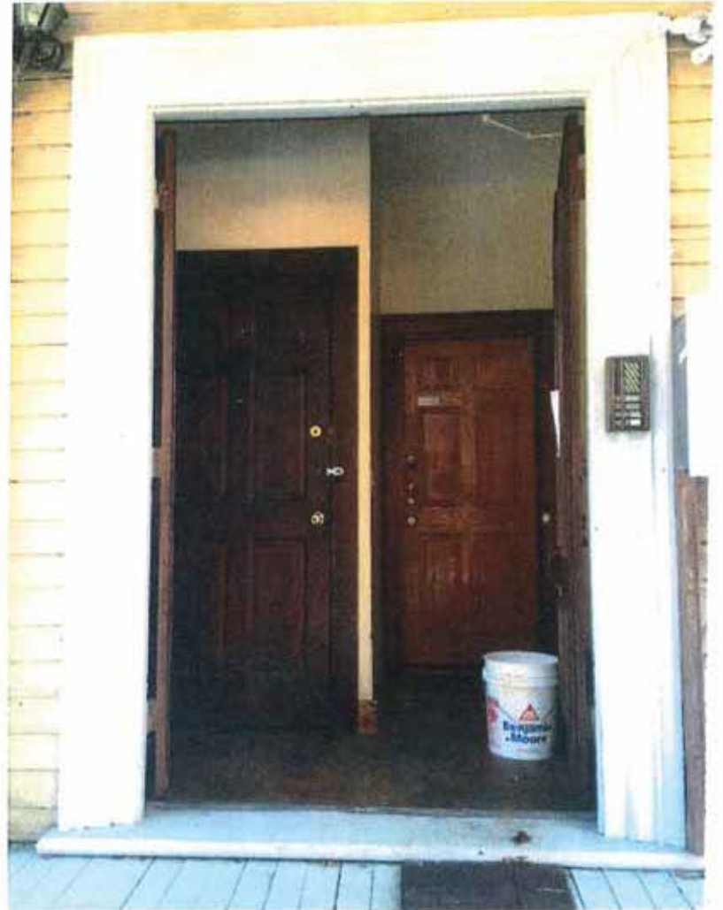
VIEW OF EXISTING ENTRY
