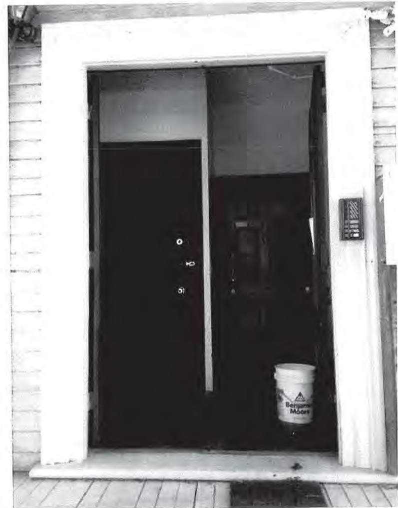
VIEW OF EXISTING ENTRY
