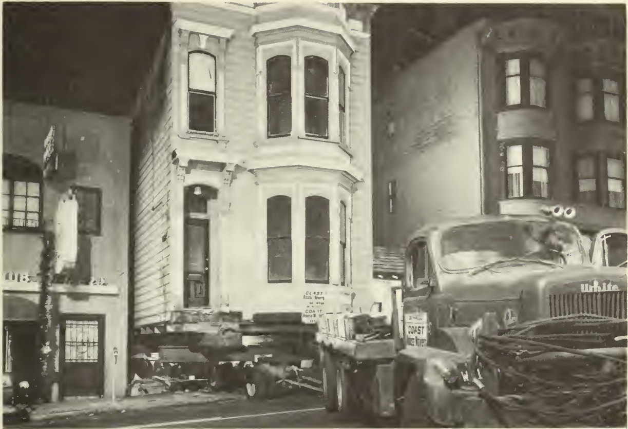
Figure 26: Housemoving in tight spaces
