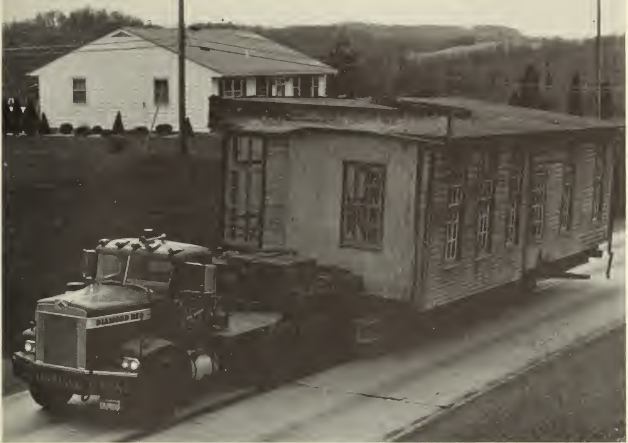
Figure 39: This section of the Gruber Wagon Works, only somewhat wider than a house trailer, was small enough to be transported over the narrow country roads on a "low-boy" flat-bed trailer. [Photograph: Courtesy of John Milner Associates]
