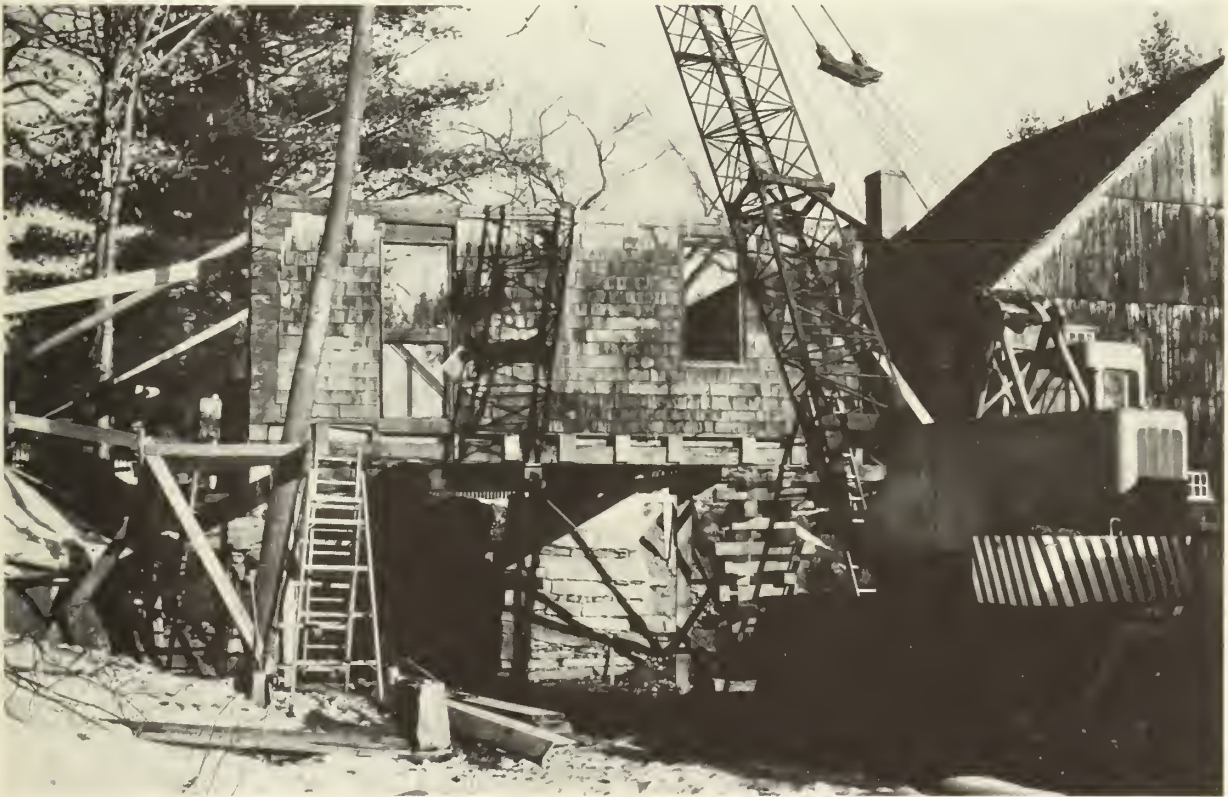
Figure 25: Using a crane to reassemble a wall unit
