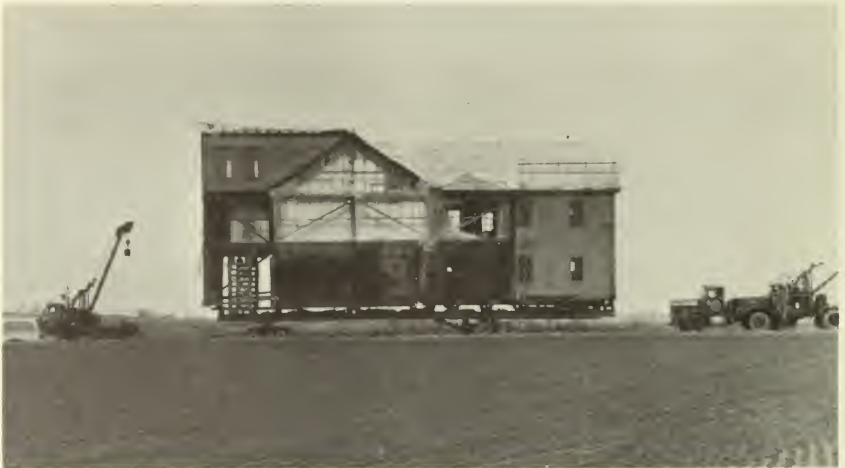
Figure 41: Temporary reinforcement for Gruber Wagon Works move
