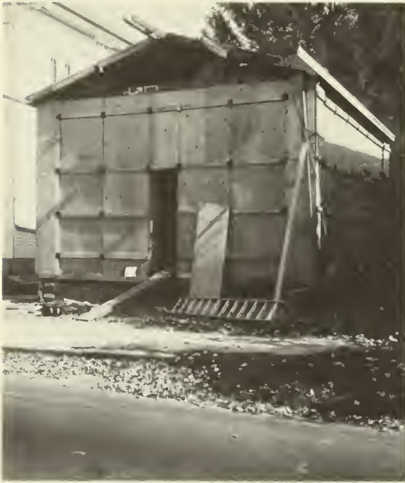
Figure 31: A protective crate for moving the Thompson Bank to Old Sturbridge Village
