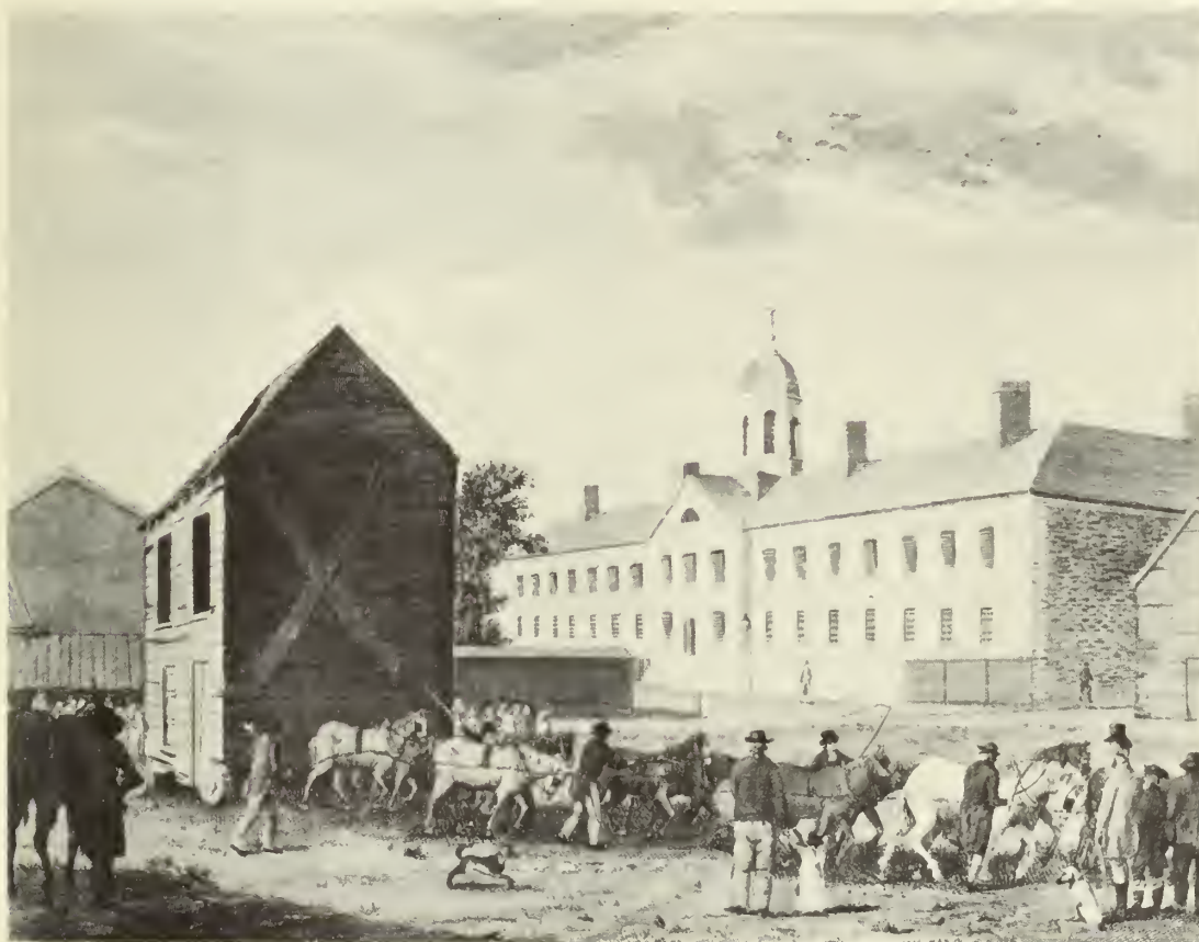
Figure 1. Moving a building in Philadelphia in 1799
