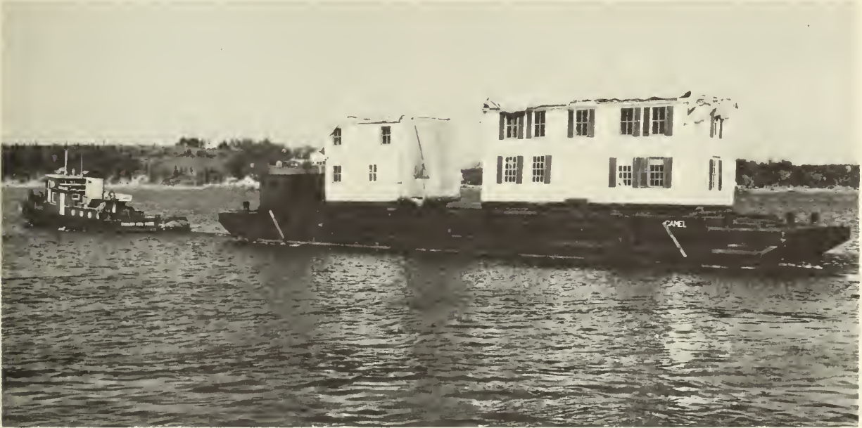
Figure 19: Moving by barge
