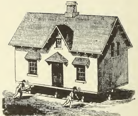
Fig. 2.—HOUSE RAISED BY SCREWS.
