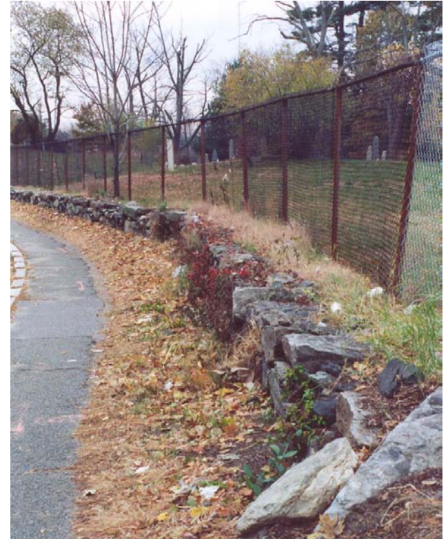
stone wall and fence along Winchester Street, South Burying Ground
