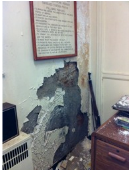
Water damage in City Hall: Above, standing water in the boiler room; at right, in a room used by Veteran's Services, plaster has fallen from a water-damaged area.
