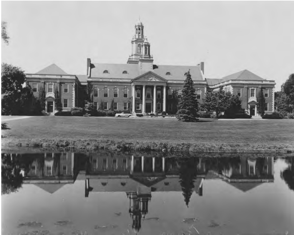
Figure 1: City Hall entry (east elevation), c.1940s. The landscape plan was designed so that the building would be mirrored in the reflecting ponds, with the reflection visible from the front steps of City Hall (Credit: Historic Newton).
