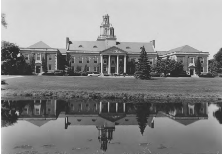
Figure 1: City Hall entry (east elevation), c.1940s. The landscape plan was designed so that the building would be mirrored in the reflecting ponds, with the reflection visible from the front steps of City Hall (Credit: Historic Newton).
