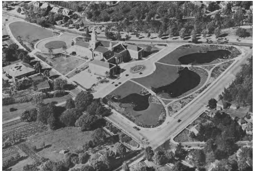
Figure 2: aerial view of City Hall and landscape after construction (Credit: Historic Newton).
