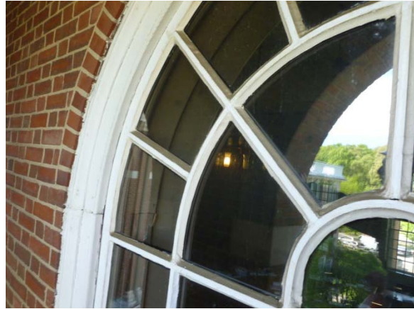
Window with sealant used as glazing putty.
