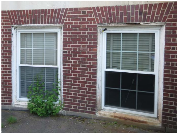
Vinyl windows installed in original wood frames
