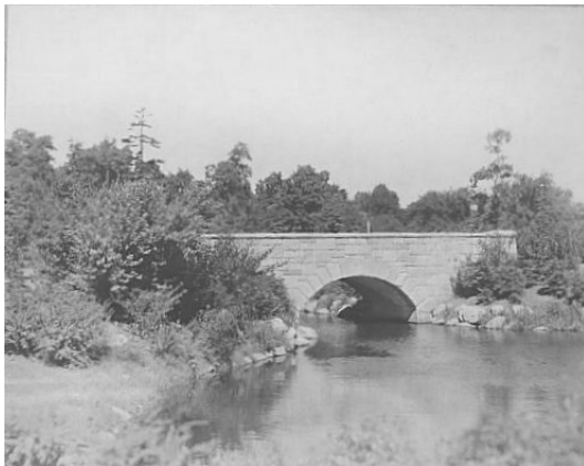
Figure 1.13. One of the rock-faced rustic bridges over the ponds in the public park, 1933 (NPS, Olmsted NHS).
