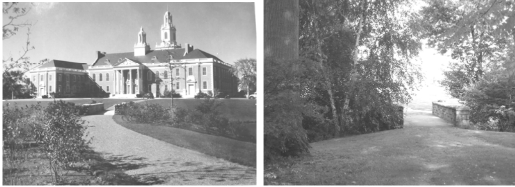
Figure 3.1. The pathway over the bridge in 1932 (NPS, Olmsted NHS) and in 2005 (Pressley Associates).
