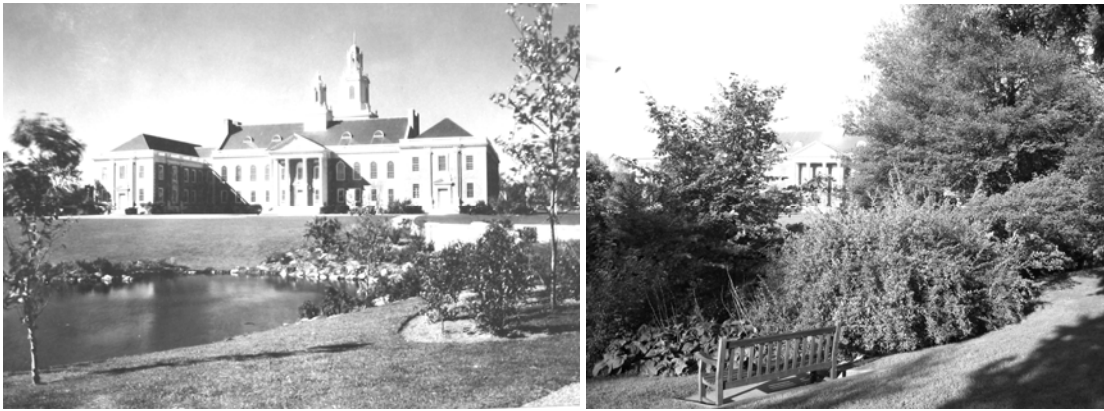
Figure 4.2. As part of the rehabilitation treatment, the original pond edges, left (NPS, Olmsted NHS), 1932, would be re-established from their current condition, right (City of Newton), 2004.
