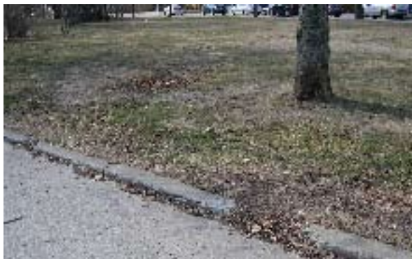
existing concrete curb at Lowell Avenue
