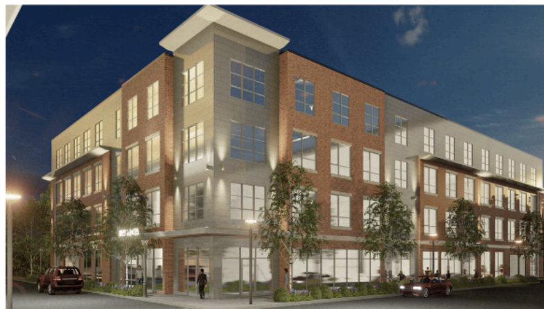
Image 1. Corner of Building 2
