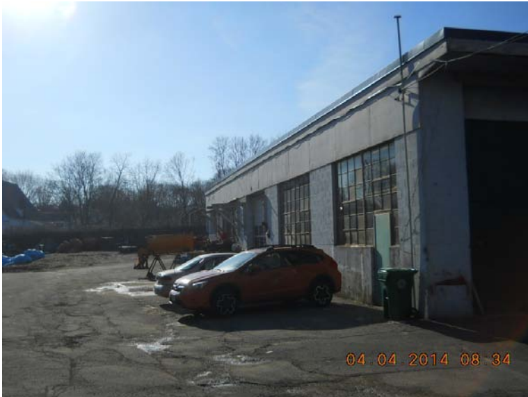
Photo #5: North face garage; UST vent pipe shown at corner building
