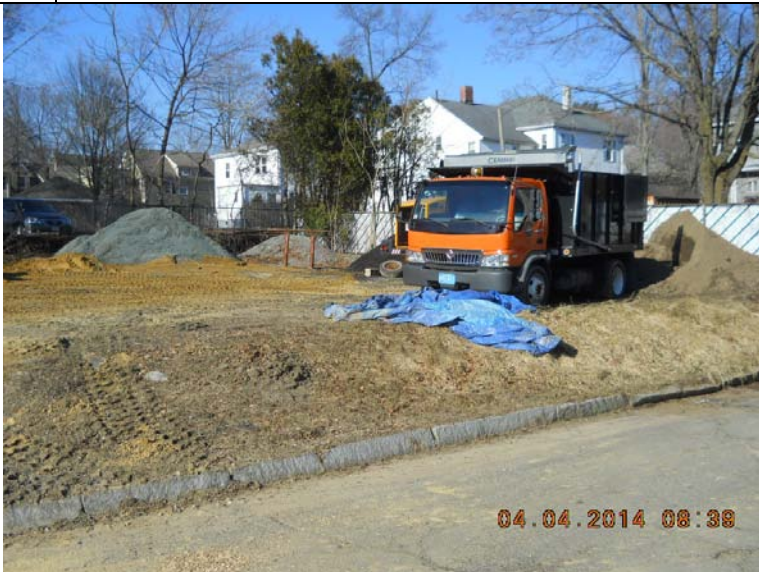
Photo #7: Sand and equipment to south of garage
