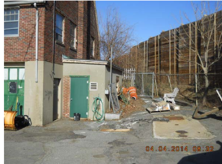
Photo #2: North side office; UST shown
