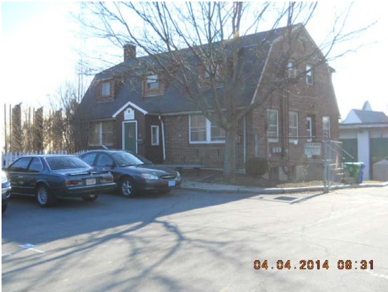
Photo #1: West face of office building
