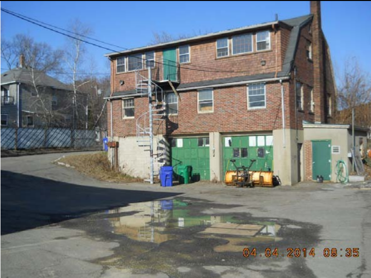
Photo #3: East face of office
