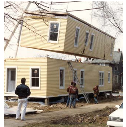
Module assembled on site.
