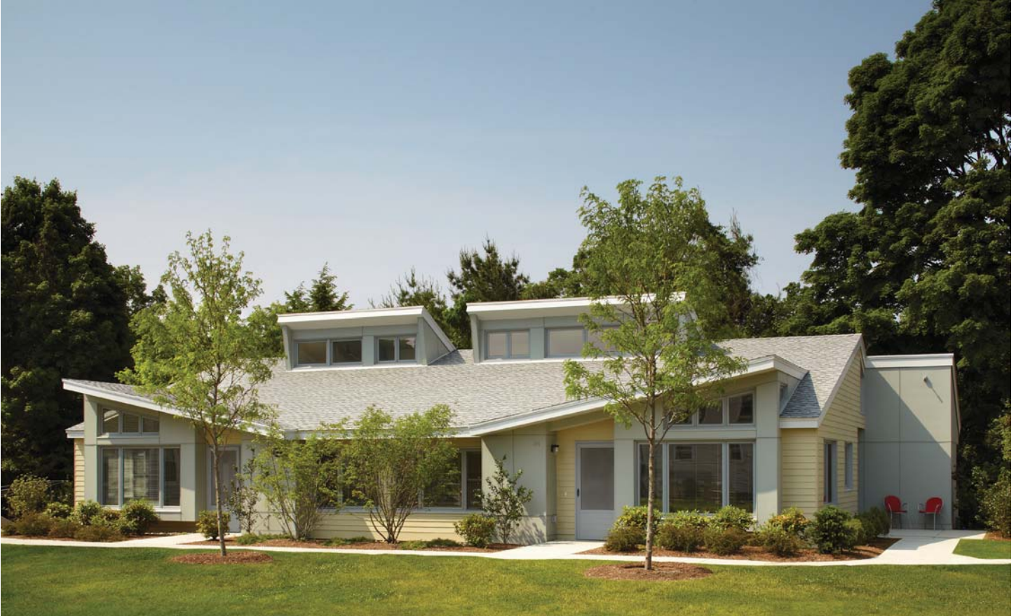
Operable windows are located to maximize natural ventilation, and passive solar heating
