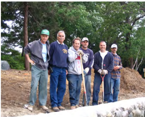
City employees work to rebuild the retaining wall in time for the 2007 beach season.
