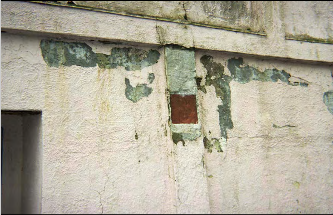
Figure 17: Exterior Bathhouse Wall - Stucco Over Clay Tile
