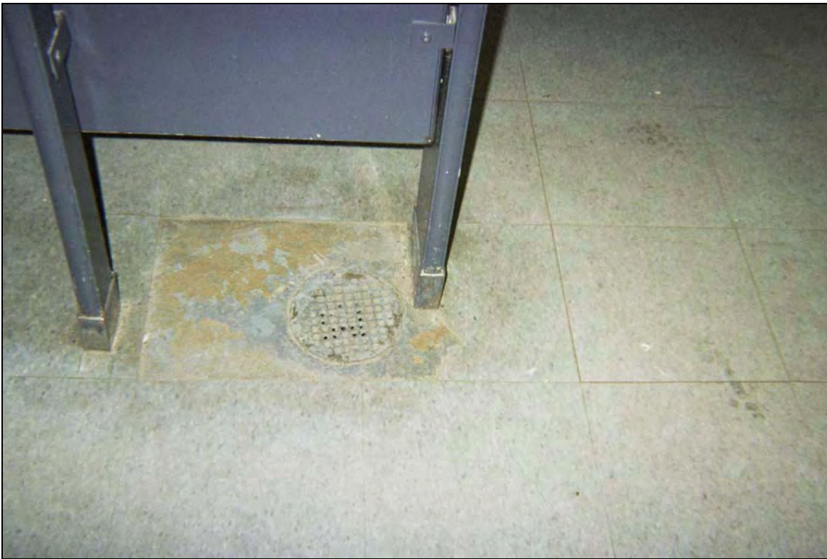
Figure 23: Interior Bathhouse - Single Floor Drain
