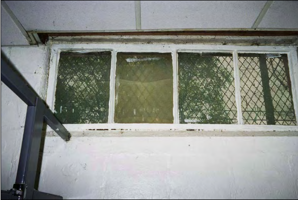
Figure 24: Interior Bathhouse - Windows
