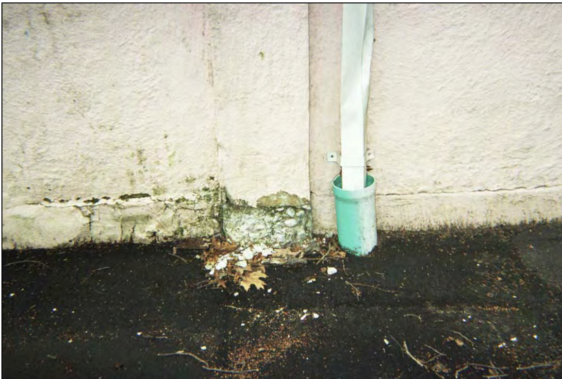
Figure 15: Exterior Bathhouse - Stucco Over Concrete Block at Ground Level
