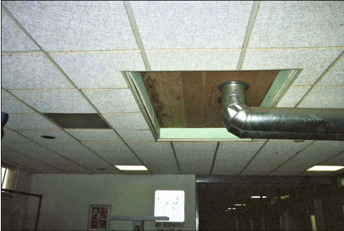
Figure 26: Interior Bathhouse - Ceiling
