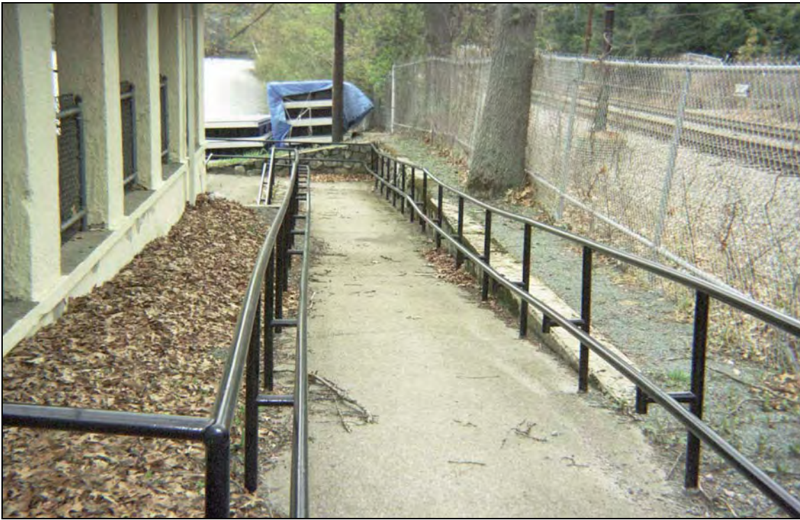
Figure 21: Exterior Bathhouse - Handicap Access Ramp Along MBTA Tracks
