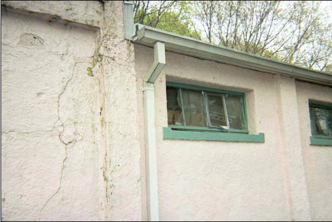
Figure 16: Exterior Bathhouse - Windows, Stucco and Roof Drainage
