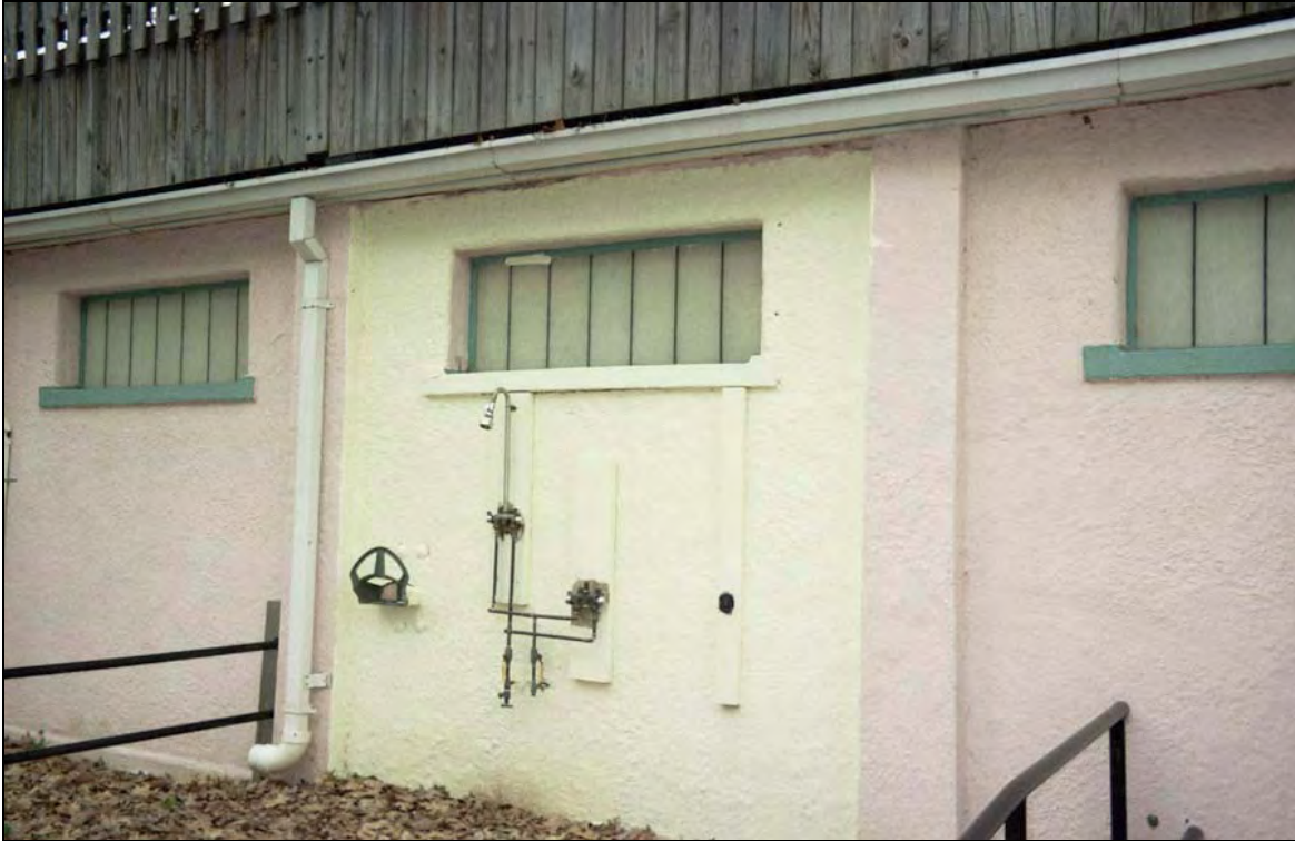
Figure 22: Exterior Bathhouse - Shower
