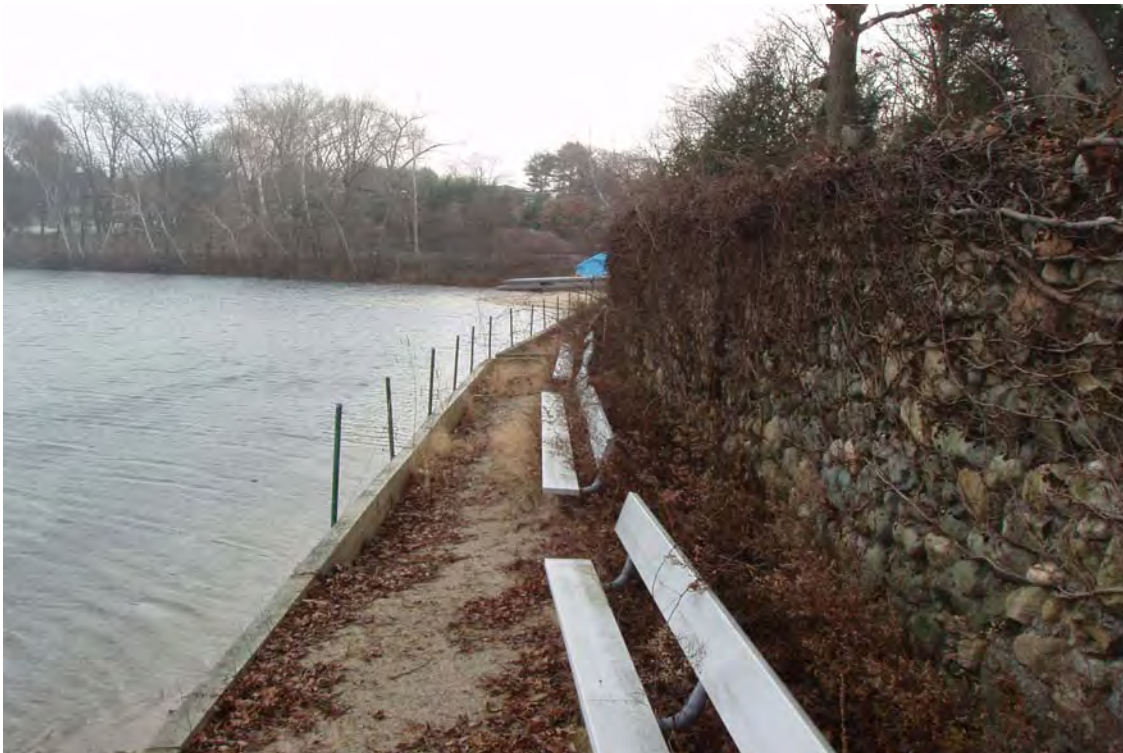
View of Retaining Wall Looking Toward City Beach
