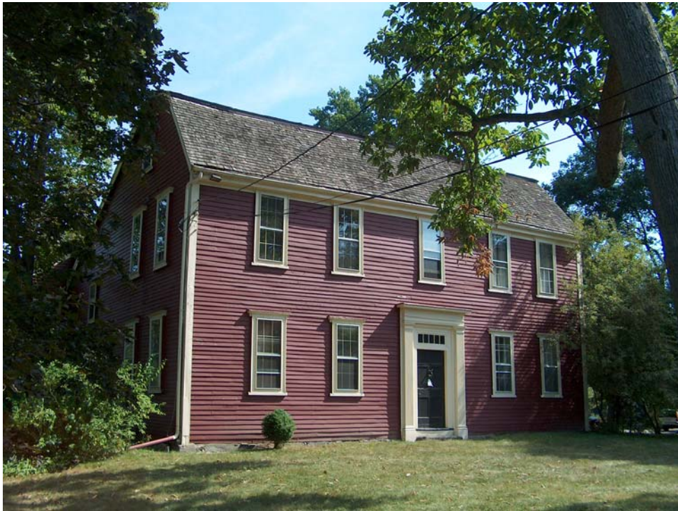
Photo A – Front Elevation of Durant Kenrick Homestead from Waverly Avenue
