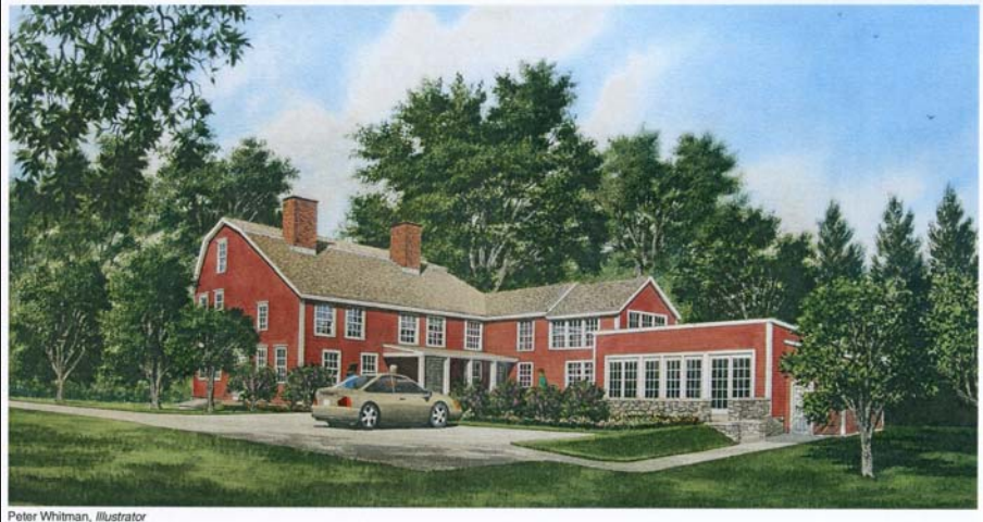
After reconstruction, view from the rear
