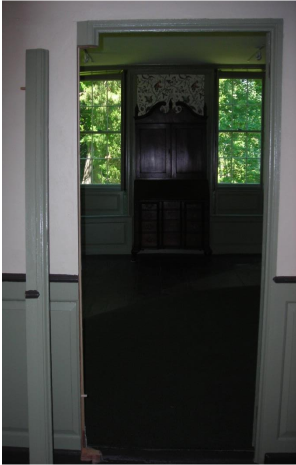
The left side of the door frame is removable to allow wheel chair passage through narrow historic doors.
