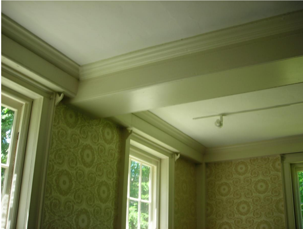
Beam installed and casings replaced
