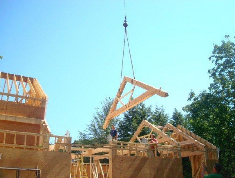
Above: roof supports being lowered into place Below: foundation for addition is poured
