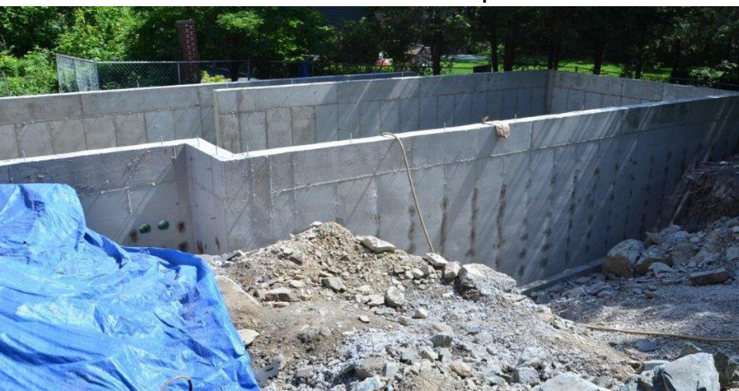
Above: roof supports being lowered into place Below: foundation for addition is poured
