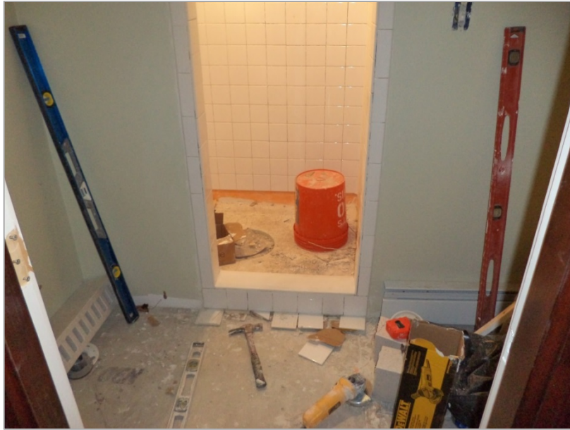
three-quarter bath added to 2 nd /3 rd floor unit
