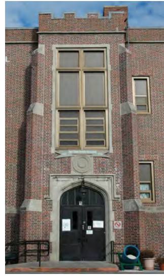
Figure 4: The front entries are given visual importance through the buttressed projection, prominent window and cast stone door surround.
