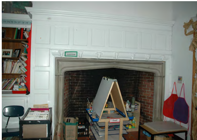
Figure 7: Fireplace in front classroom with stone surround and carved wood mantel.
