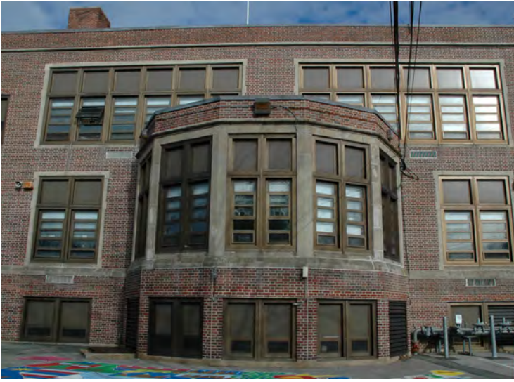
Figure 3: The windows of the front projection and of the general façade, although severely altered and far less elegant, retain vestiges of their original configuration in the wider horizontal mullion dividing the transom sashes from the lower sashes. Compare to the historic photo in figure 1.
