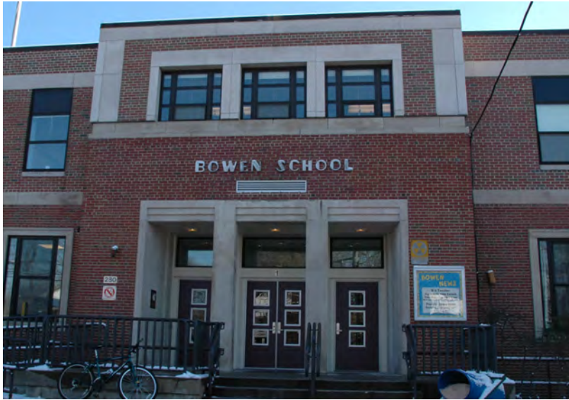
Figure 1 (top): main entrance
