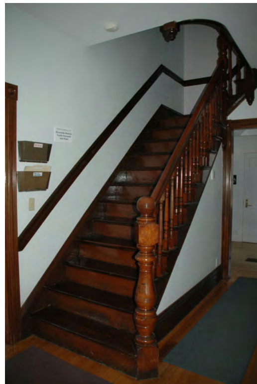
Figure 6: Original interior staircase in good condition.
