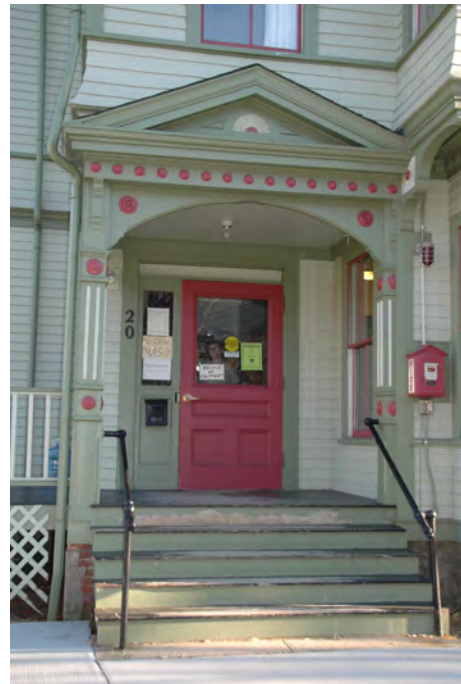
Figure 4: Ornamented front porch with a new accessible ramp added to side.
