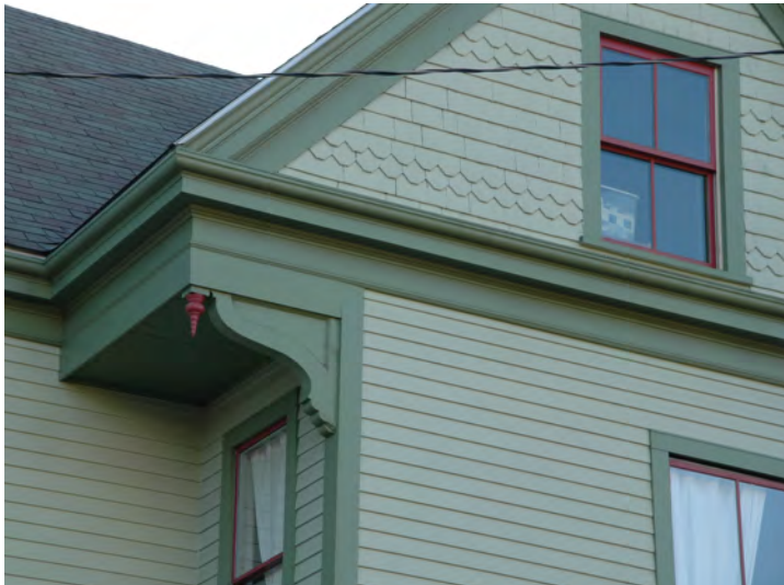
Figure 3: Decorative exterior details include brackets with finials, supporting the roof edges and patterned shingles at the gable ends.
