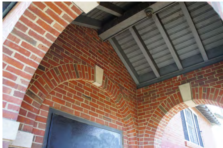
Figure 5: The rounded arch doorways with cast stone keystones and springline are also present within the pavilions. Note also the painted beadboard ceiling and rafters in the lower east corner.
