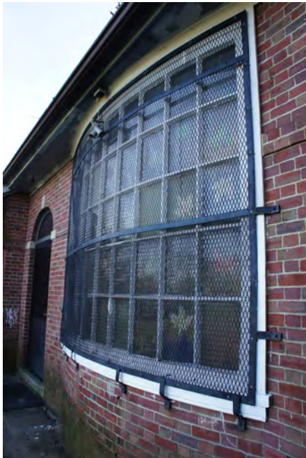
Figure 4: the original 45-pane wood bow Window at the center of the north façade is still intact, although covered with a metal grate.
