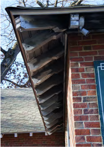
Figure 2: the prominent roof overhang with a wood fascia and beadboard sheathing is supported by rafter tails that wrap the corners of the roof.
